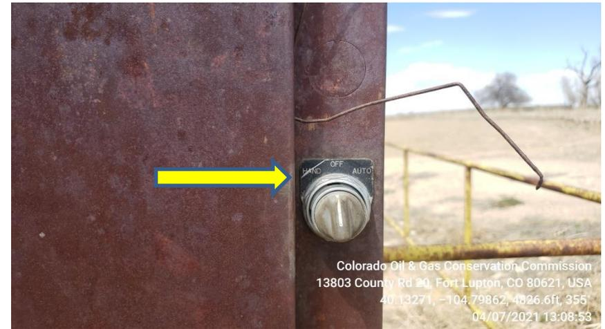
Photo 11 Electric panel is shut off .
