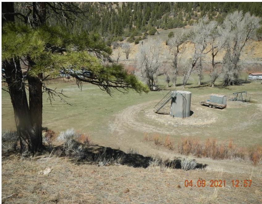
View of AST used by Chavez #1 and #2 wells.
