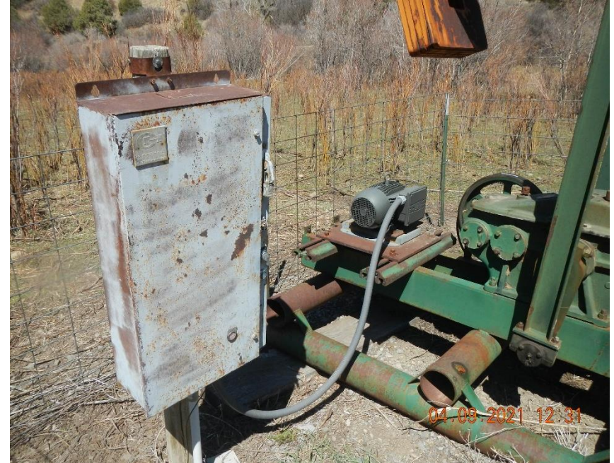
Electrical supply to pump jack turned off during this inspection.
