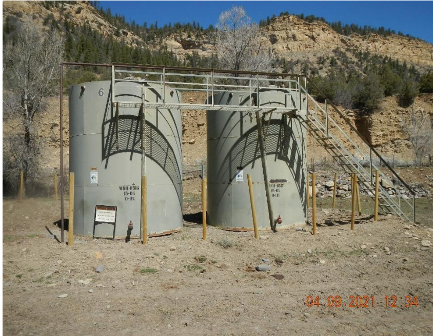
Albert Martinez #1 tank battery. Anchors were observed during this inspection. Tanks are not attached to anchors.
