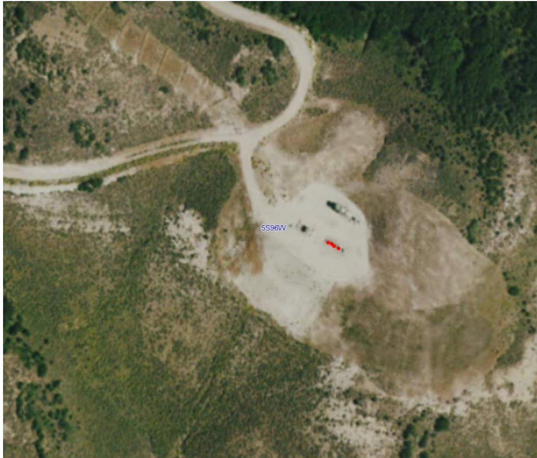
Photo 8: 2019 COGIS aerial imagery. Photo shows areas on the south end of the Location where topsoil does not appear to have been replaced in accordance with 1003.e.(2).
