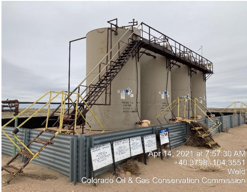
Photo #3 Tank Battery
