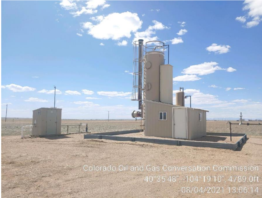
Photo 3 – Heater Treater
