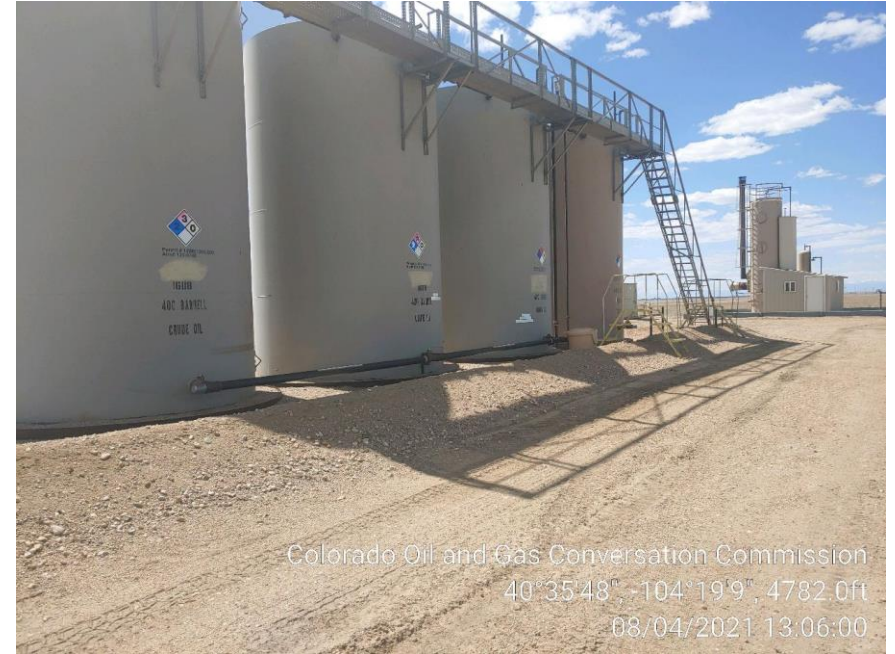
Photo 4 – Tank Battery
