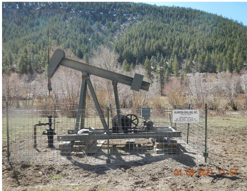
Nielson #4 well head, pump jack, and location sign. Location sign does not meet the requirements of Rule 605.d(1).
