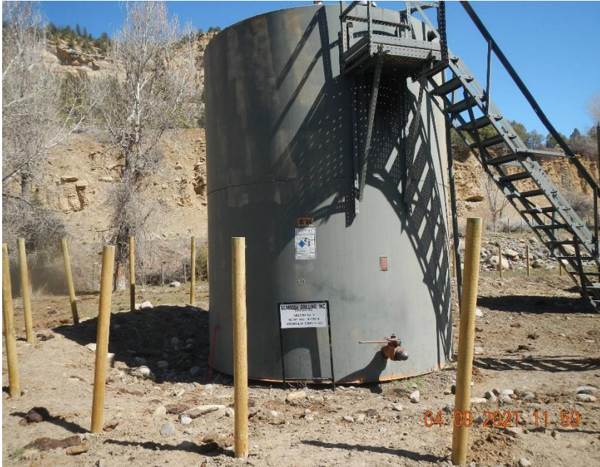
300 bbl. steel AST for Nielson #4. Stained soil at load out valve. Battery sign is non-compliant.
