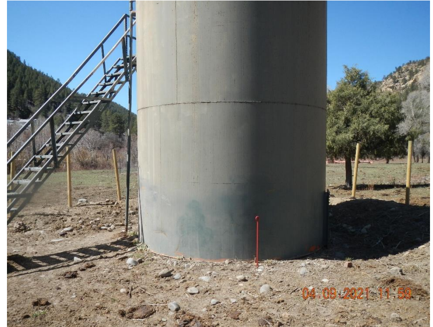
Anchor observed during this inspection. Tank is not anchored.
