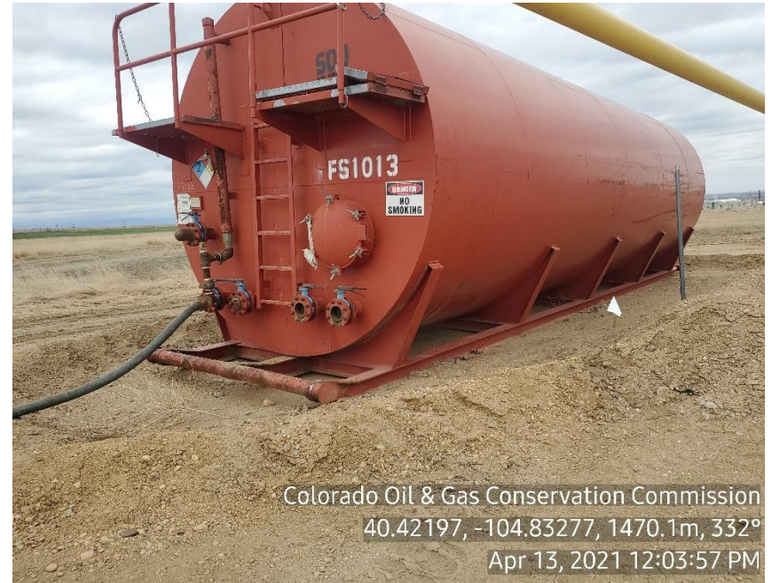
Photo 8: Tank not grounded
