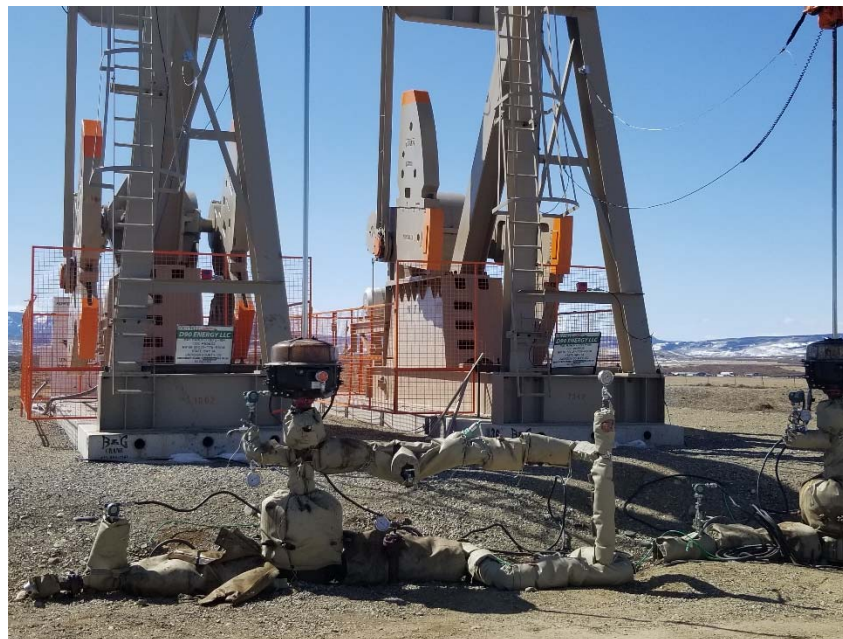
Photo 4. Wellhead signs without all necessary information.
