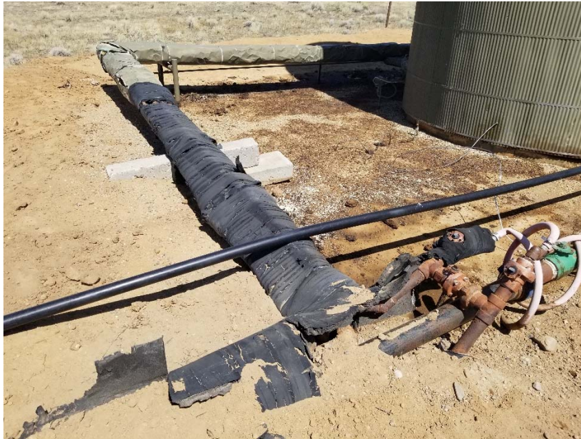
Photo 1. Fluid removed. Stained soil remains. Unconsolidated material used in attempted berm repair.
