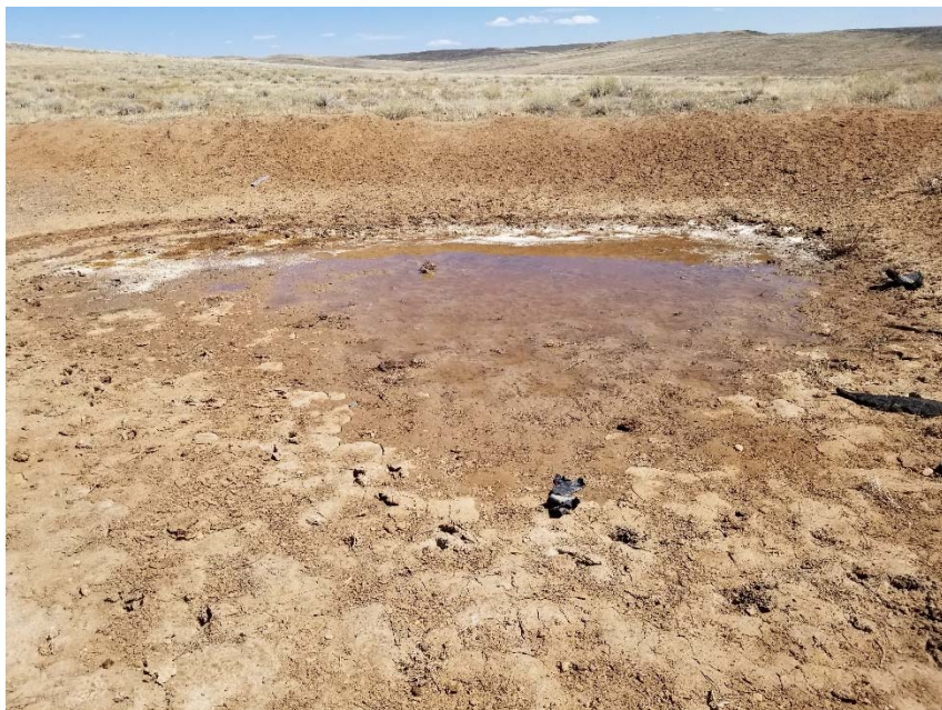
Photo 5. Fluid and stained soil in north side of berm.
