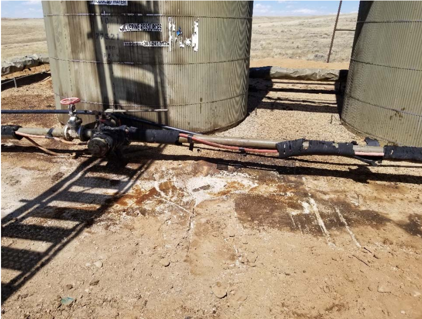
Photo 3. Leak stopped. Fluid removed. Stained soil remains.
