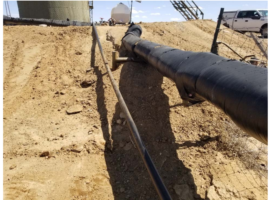
Photo 2. Unconsolidated material used in attempted berm repair. Stained soil.
