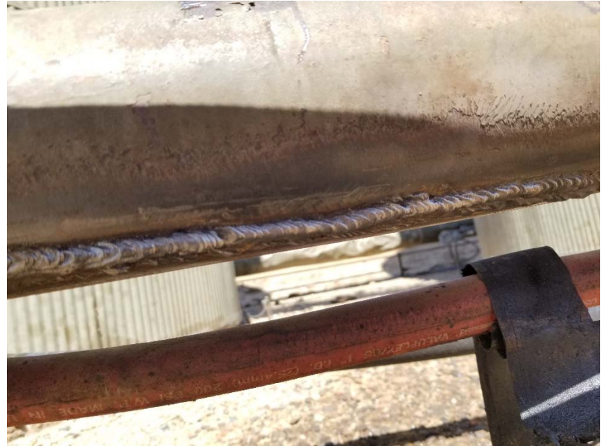
Photo 4. Fresh weld in apparent “repair” of flowline where leak was occurring.
