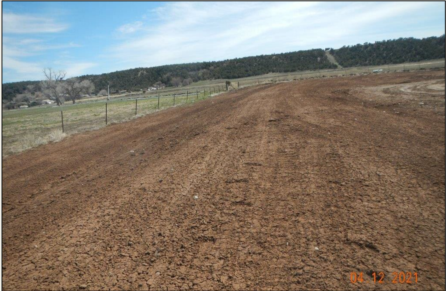
Photo 2. View of the northern project area from the northwestern corner facing eastward. Revegetation is conducted within the interim reclamation areas. Germination observed. However, bare soils are not protected and erosion controls not installed.
