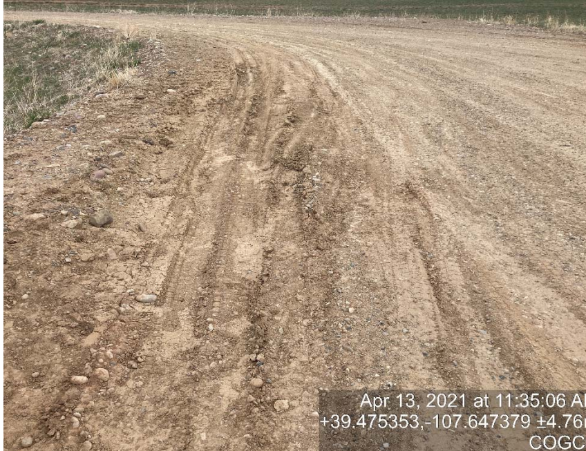
Lack of stabilization/compaction
