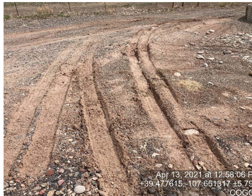
Lack of stabilization/compaction
