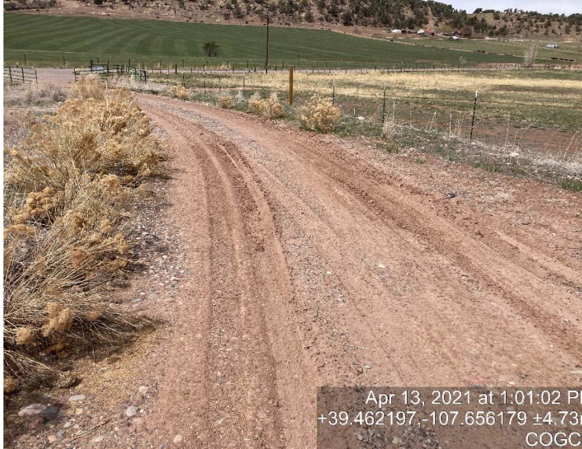
Lack of stabilization/compaction
