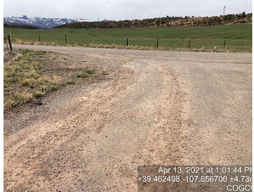
Lack of stabilization/compaction/sediment moving off of location
