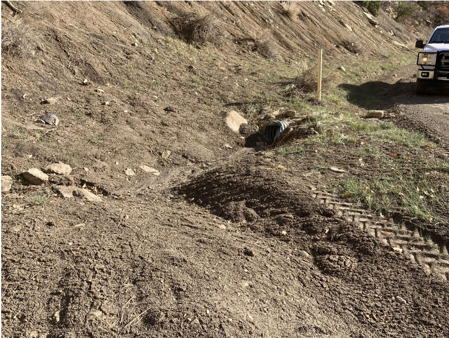
PHOTO 2: THE SEDIMENT ACCUMULATION WAS REMOVED FROM THE CULVERT INLET THAT INTERCEPTS THE AROYO ON THE CUT SLOPE AND IS UP GRADIENT OF THE INTERSECTION BELOW. THE BAR DITCH WAS DOMINATED TO DIRECT RUN OFF FROM THE LEASE ROAD TOWARD THE CULVERT INLET.
