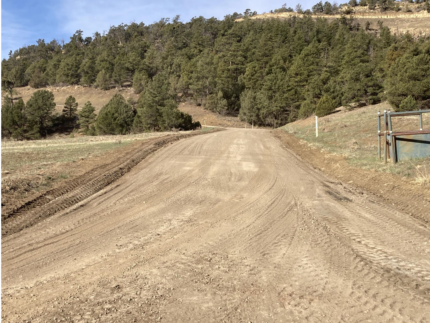
PHOTO 1: THE ROAD SURFACE WAS CROWNED TO CREATE SHEET FLOW AND ELIMINATE THE TIRE RUTS AND SURFACE EROSION. ADDITIONAL GRAVEL WAS ADDED TO THE ROADWAY SURFACE FOR STABILIZATION UP TO THE HIWAY 12 FACING SWITCH BACK. THE BAR DITCH WAS RECONFIGURED TO ELIMINATE THE EROSION.
