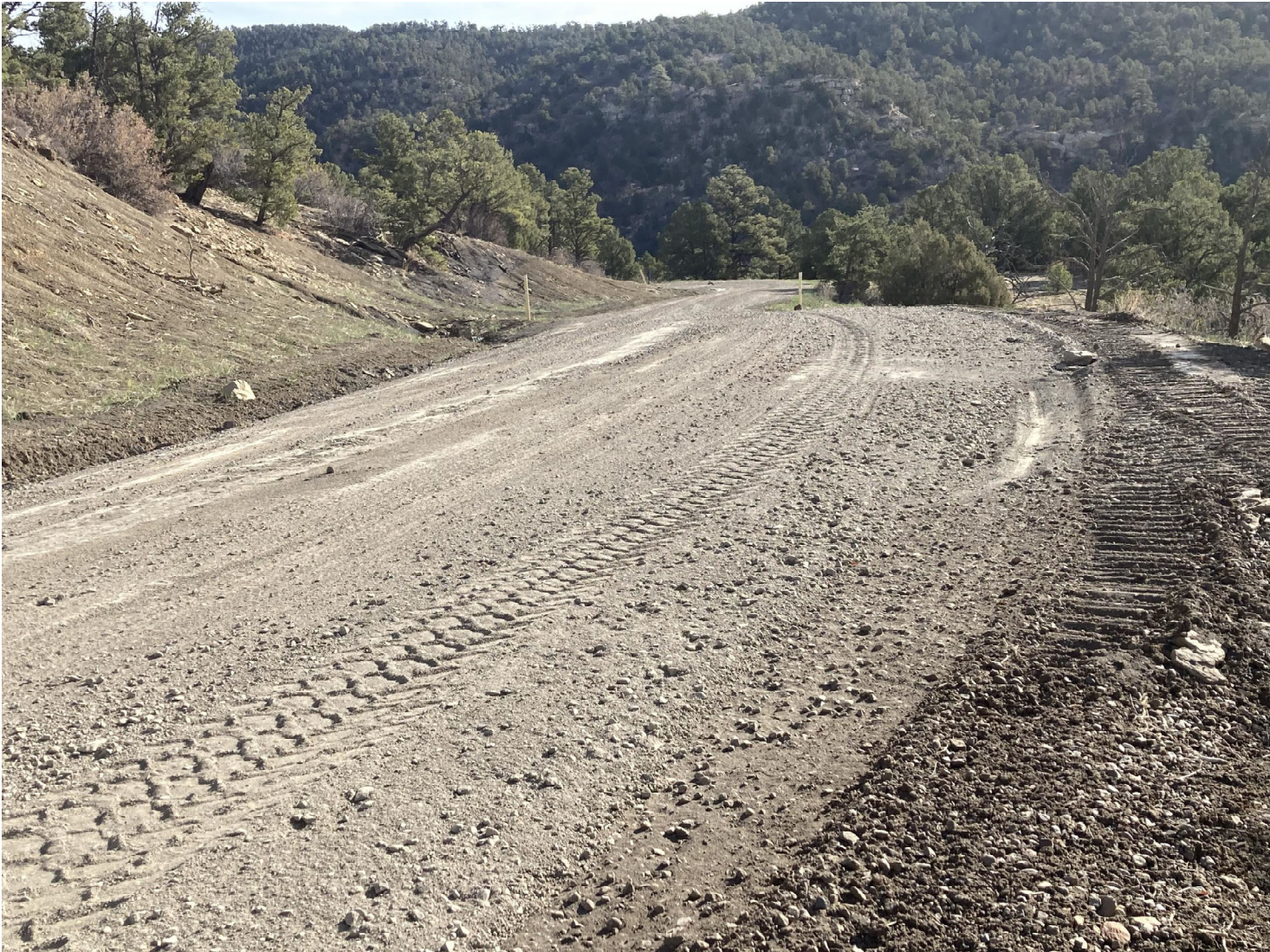
PHOTO 6: THE ROAD SURFACE WAS CROWNED TO CREATE SHEET FLOW. ADDITIONAL GRAVEL WAS ADDED TO THE ROADWAY SURFACE FOR STABILIZATION. THE BAR DITCH WAS DOMINATED TO DIRECT STORMWATER TO THE CULVERT INLET
