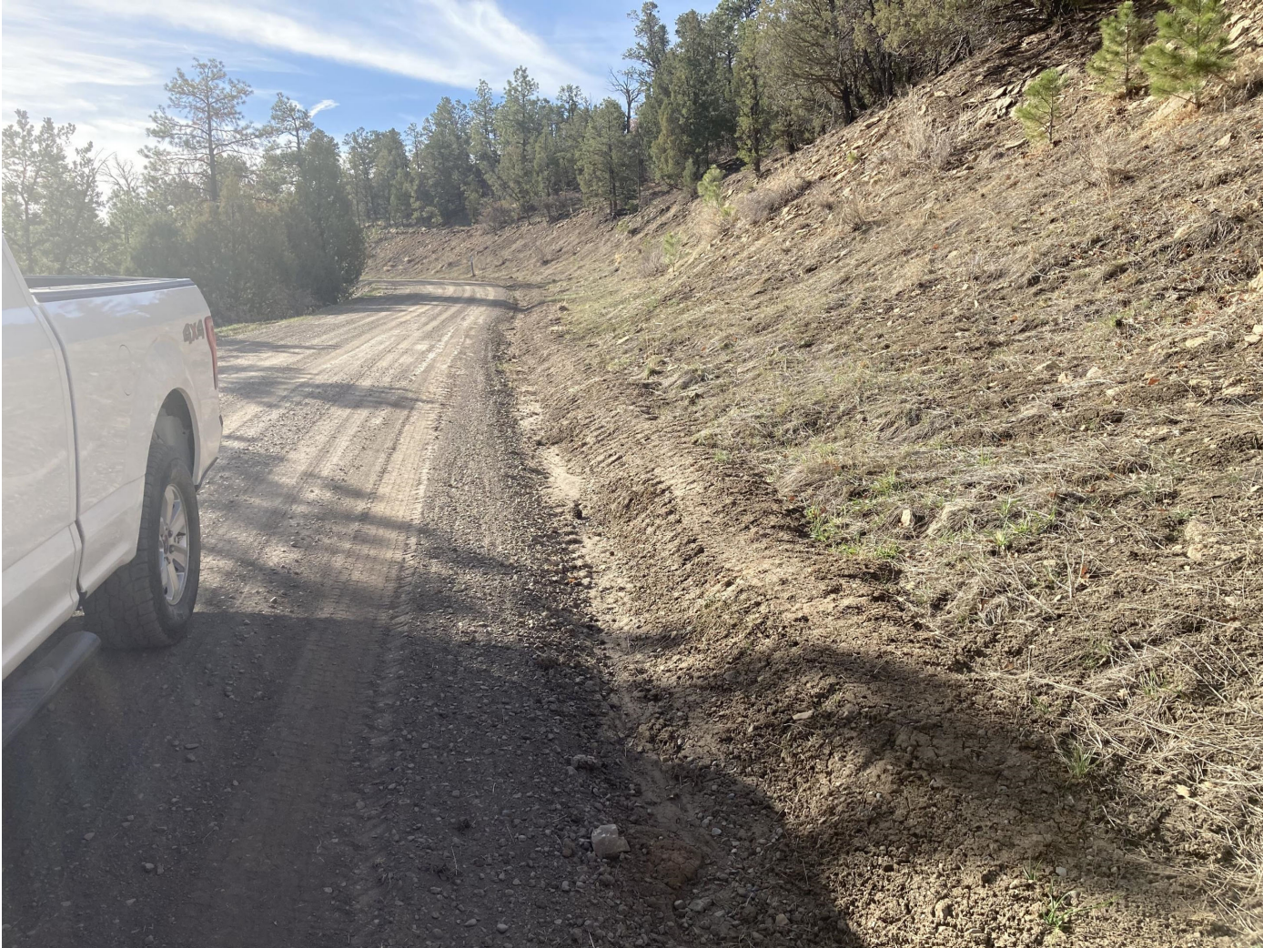
PHOTO 10: THE BAR DITCH WAS DOMINATED TO RECEIVE STORMWATER RUN OFF FROM THE LEASE ROAD.
