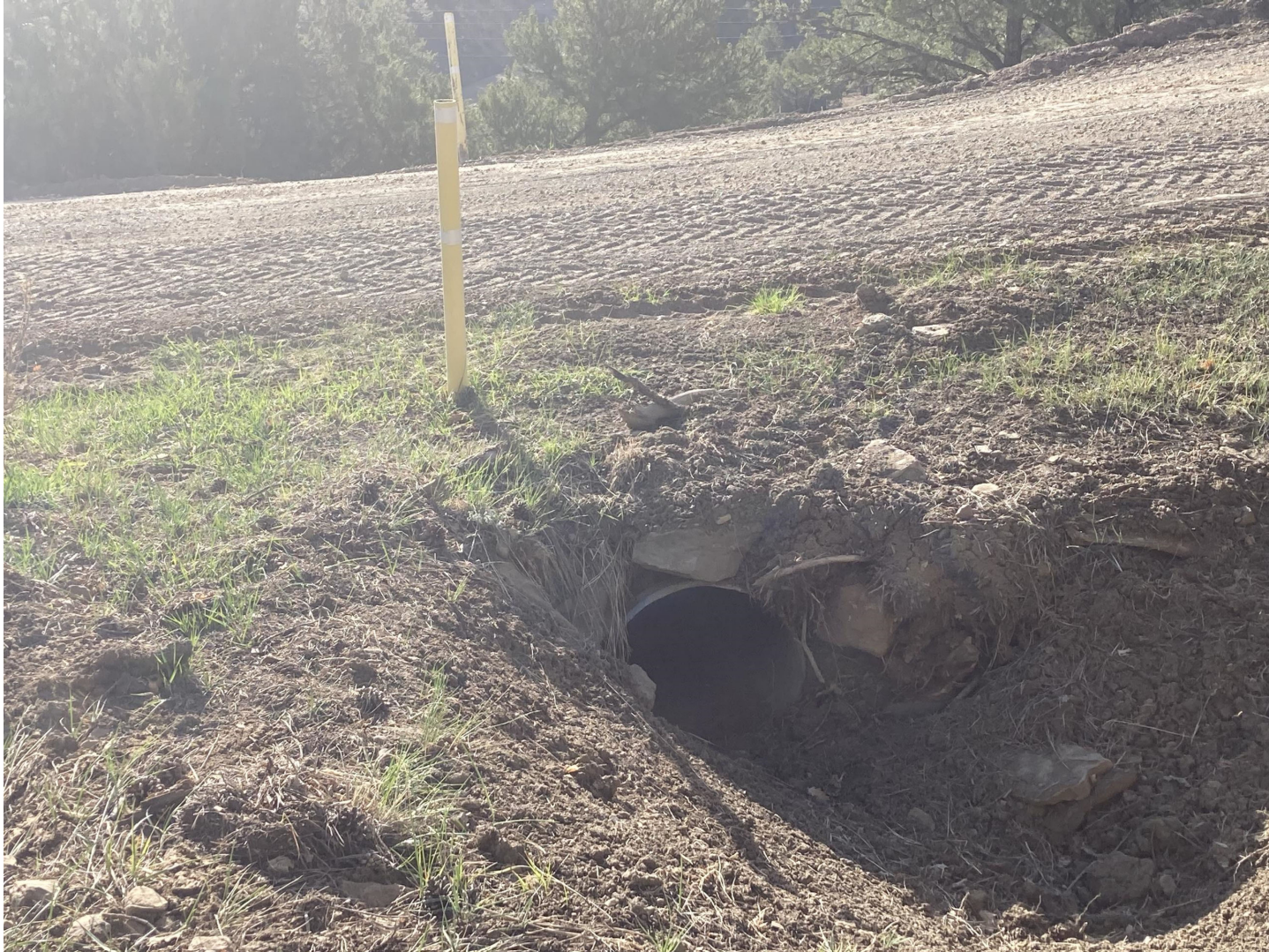
PHOTO 5: THE SEDIMENT ACCUMULATION WAS REMOVED FROM THE CULVERT INLET
