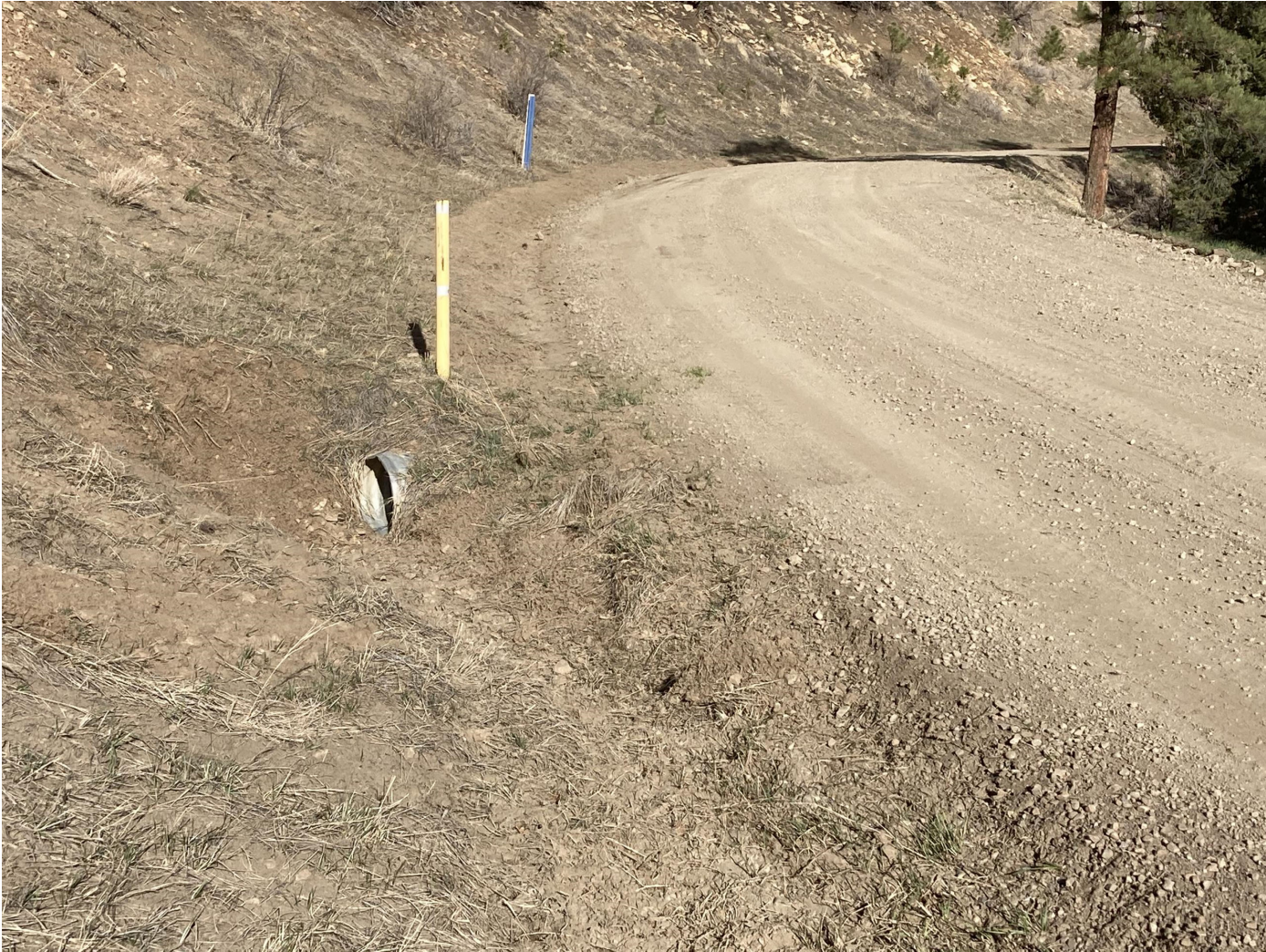
PHOTO 9: THE SEDIMENT ACCUMULATION WAS REMOVED FROM THE CULVERT INLET
