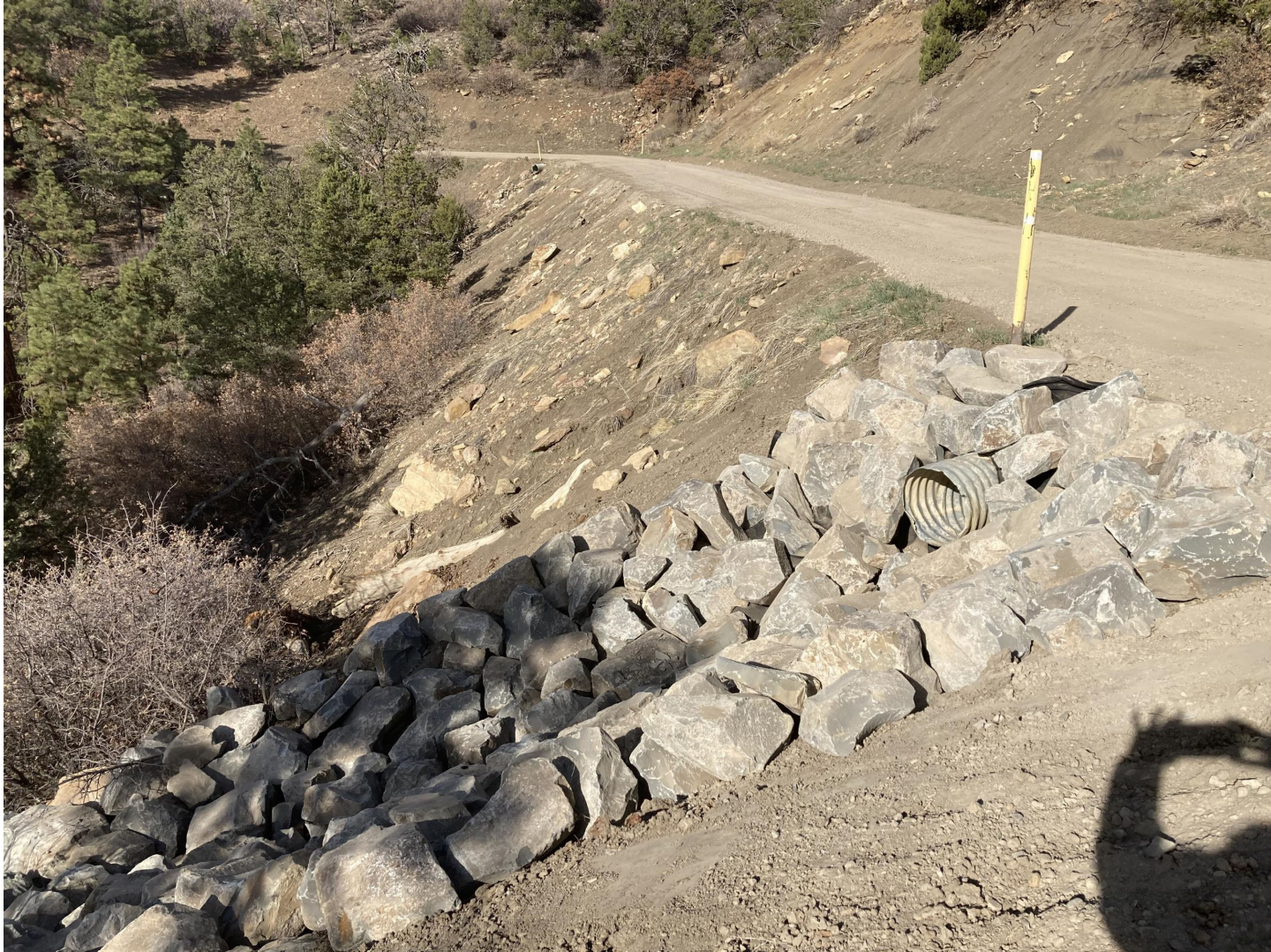
PHOTO 4: THE EROSION ON THE CULVERT OUTLET WAS CORRECTED AND ARMOR WAS INSTALLED FOR EROSION CONTROL.
