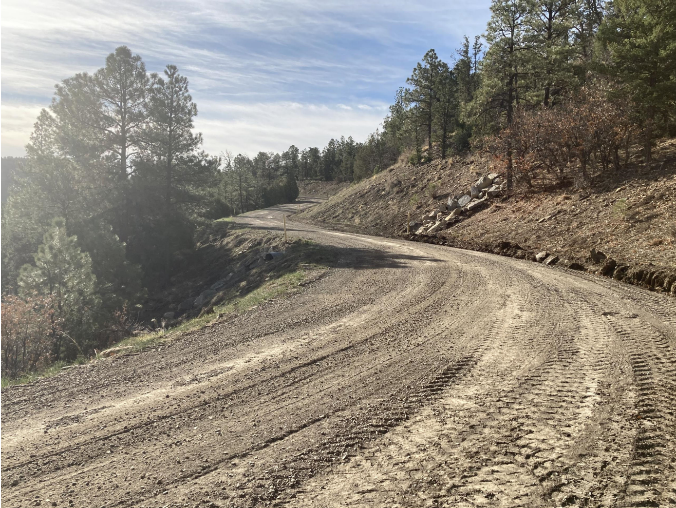
PHOTO 8: THE ROAD SURFACE WAS CROWNED TO CREATE SHEET FLOW. ADDITIONAL GRAVEL WAS ADDED TO THE ROADWAY SURFACE FOR STABILIZATION. THE BAR DITCH WAS DOMINATED TO DIRECT STORMWATER TO THE CULVERT INLET
