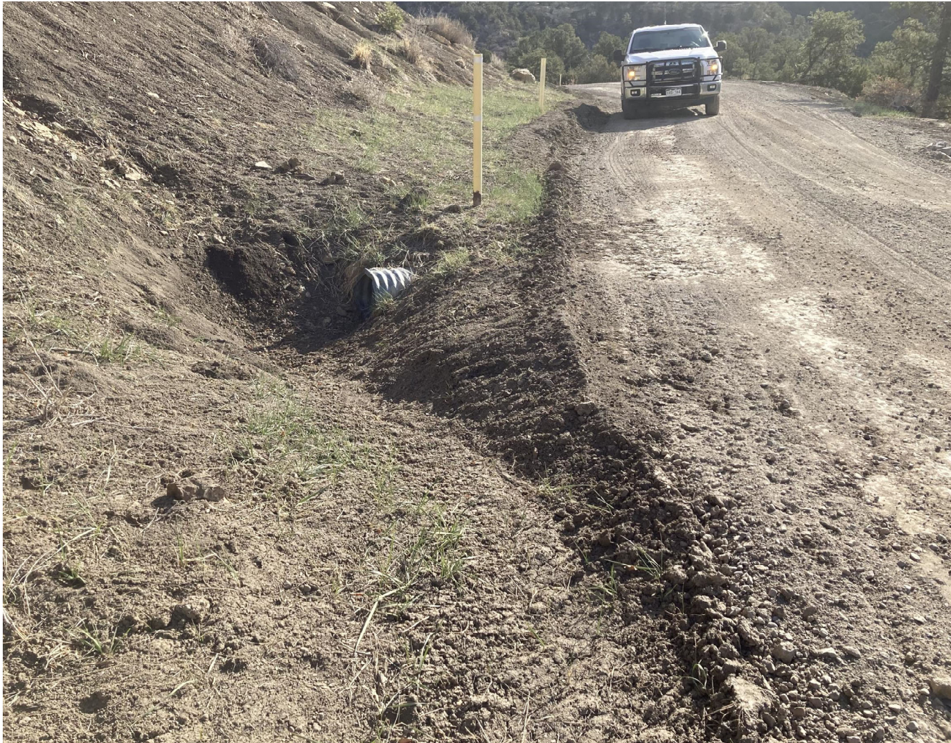
PHOTO 7: THE SEDIMENT ACCUMULATION WAS REMOVED FROM THE CULVERT INLET
