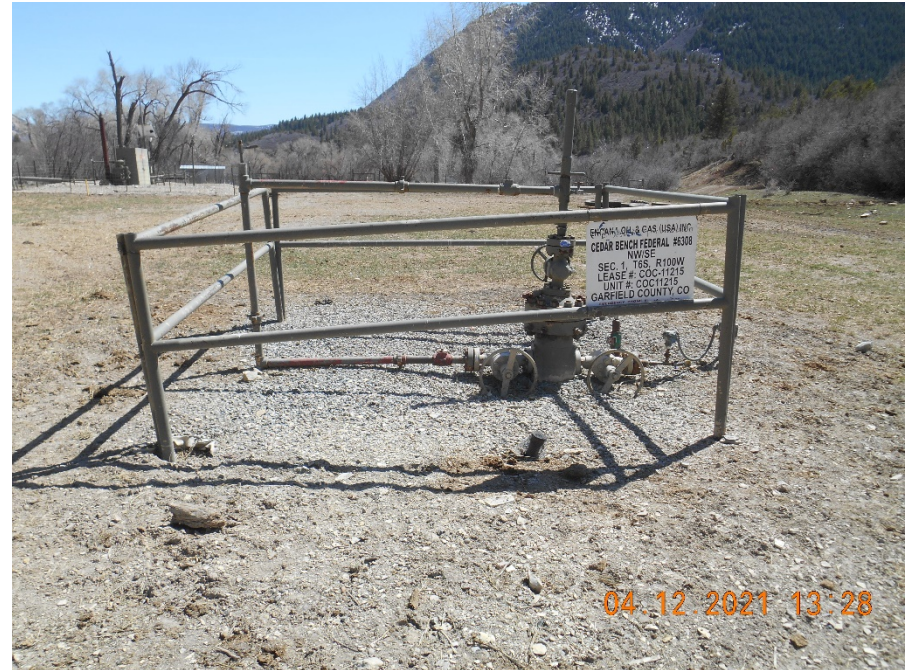
Wellhead with fence and sign
