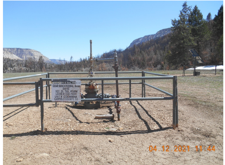
Wellhead with fence and sign
