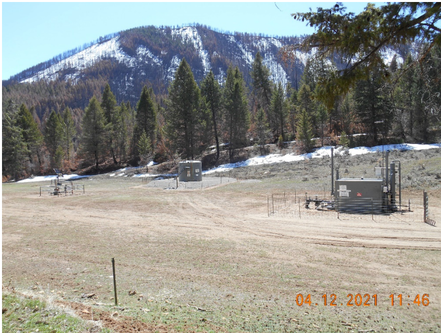
Location overview looking S
