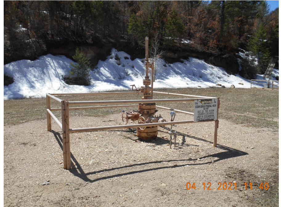
Wellhead with fence and sign
