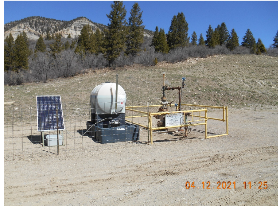
Wellhead with fence and sign
