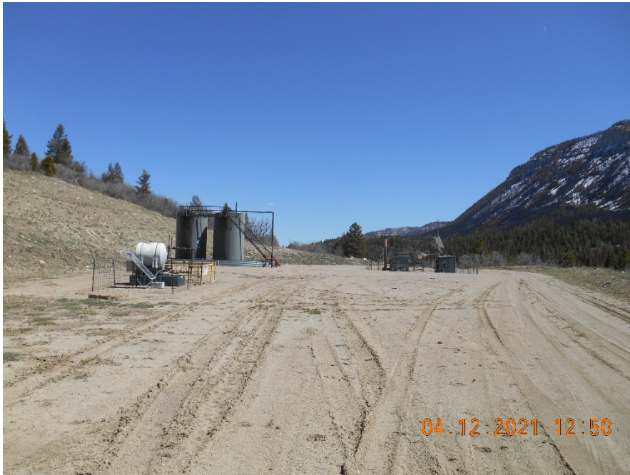
Location overview looking E
