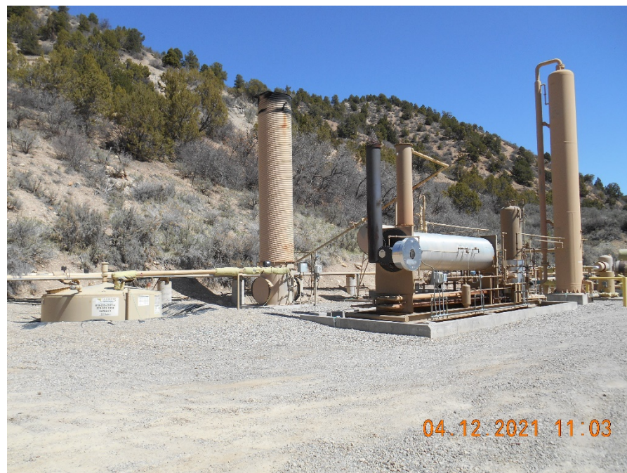
Separator, Dehydrator and combustor for compressor facility
