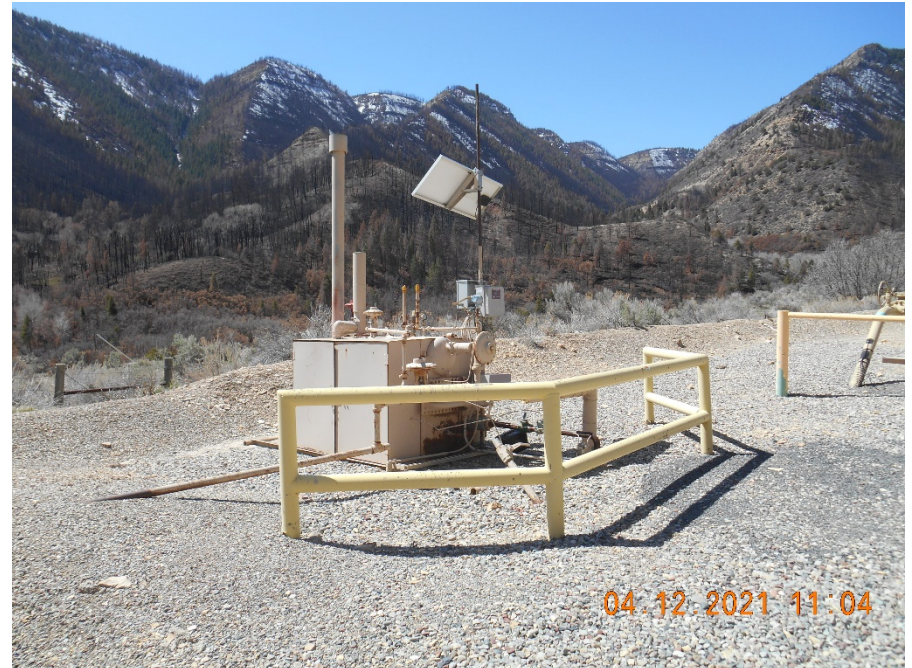
Separator with pipe barricade
