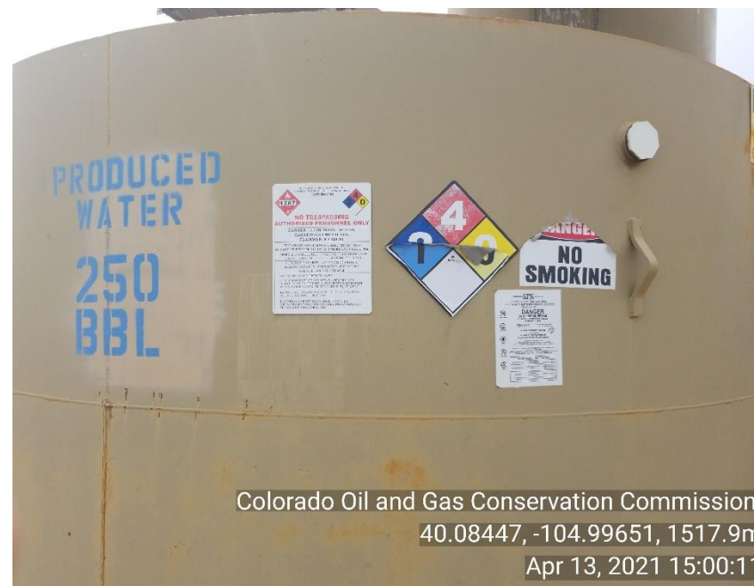
Photo 10 NFPA placard peeling and faded on produced water tank.
