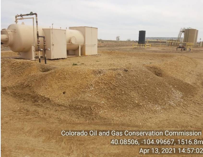
Photo 5 Secondary BMP in disrepair Prairie dog holes.
