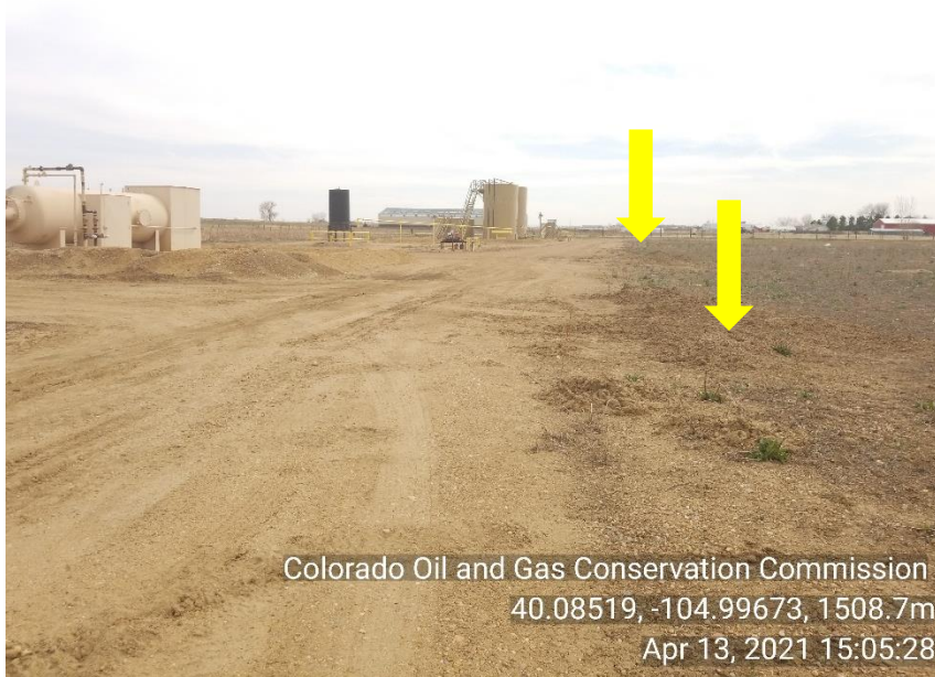
Photo 13 Material being pushed off location not NO BMP's in place.
