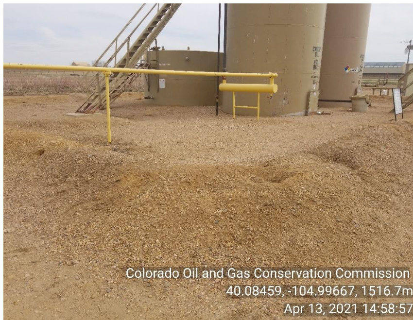
Photo 7 Secondary containment in disrepair.
