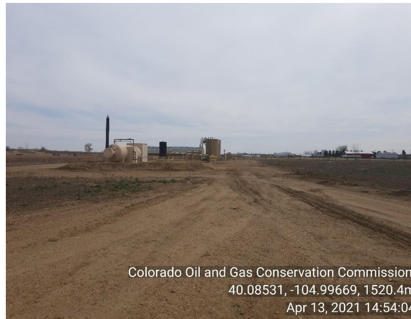
Photo 2 production equipment. Ruts on road and location no BMP's.
