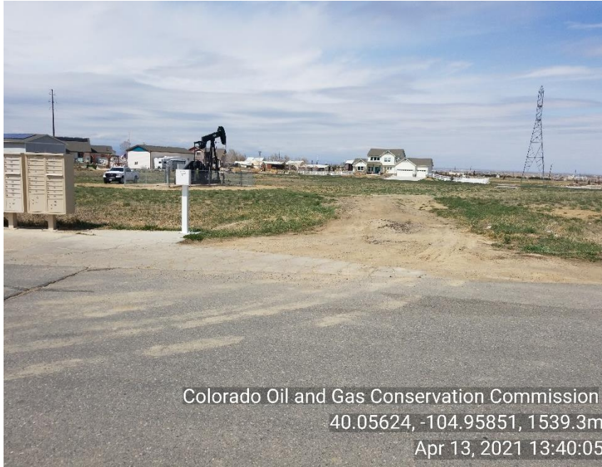
Photo 3 Tracking pad: No BMP in place tracking sediment on to public road.
