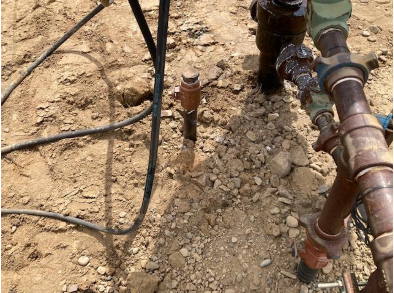
CAPPED THIS LINE SO BRADENHEAD PRESSURES CAN BE MONITORED to comply with Rule 341.
