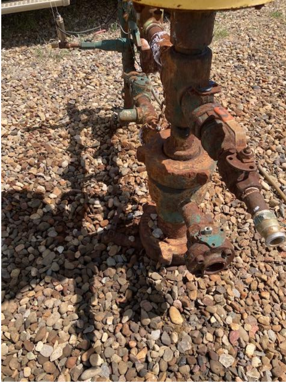
Plumbed Bradenhead to surface to comply with Rule 341.
