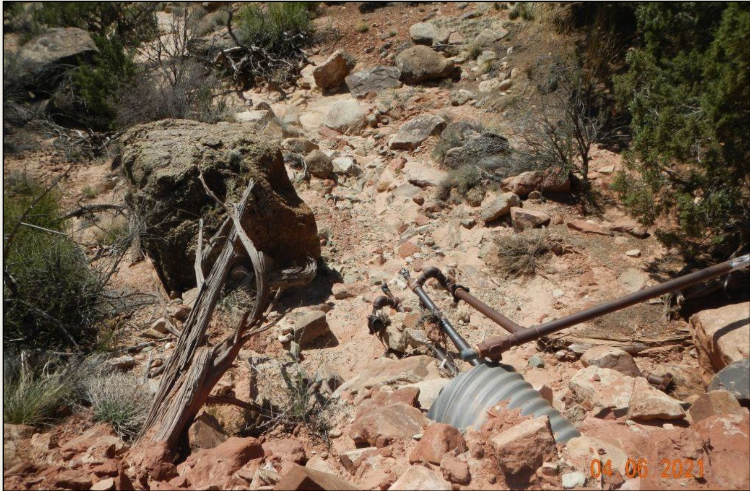
Photo 12. View of flowline at drainage intersection. Valve is open into drainage.
