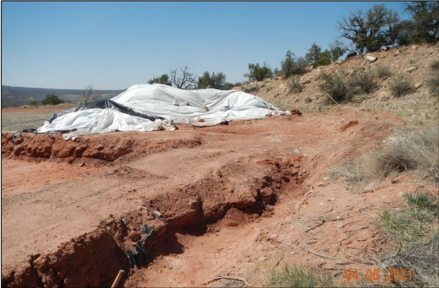
Photo 9. View of covered soil pile in the western project area.
