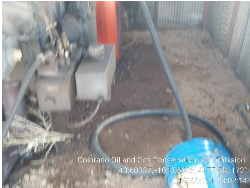
Photo 9 – Stained Soil at Gas Engine
