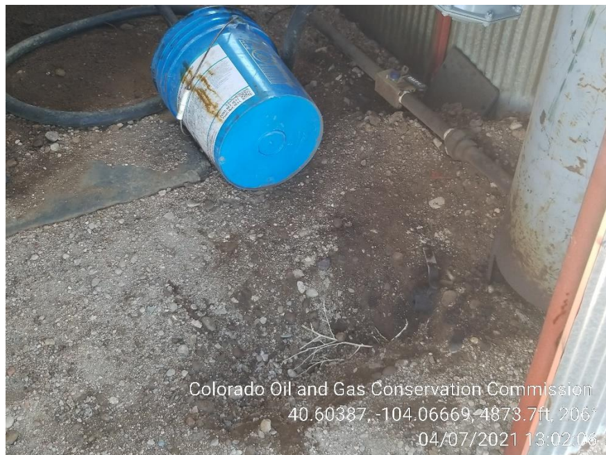
Photo 7 – Stained Soil at Gas Engine
