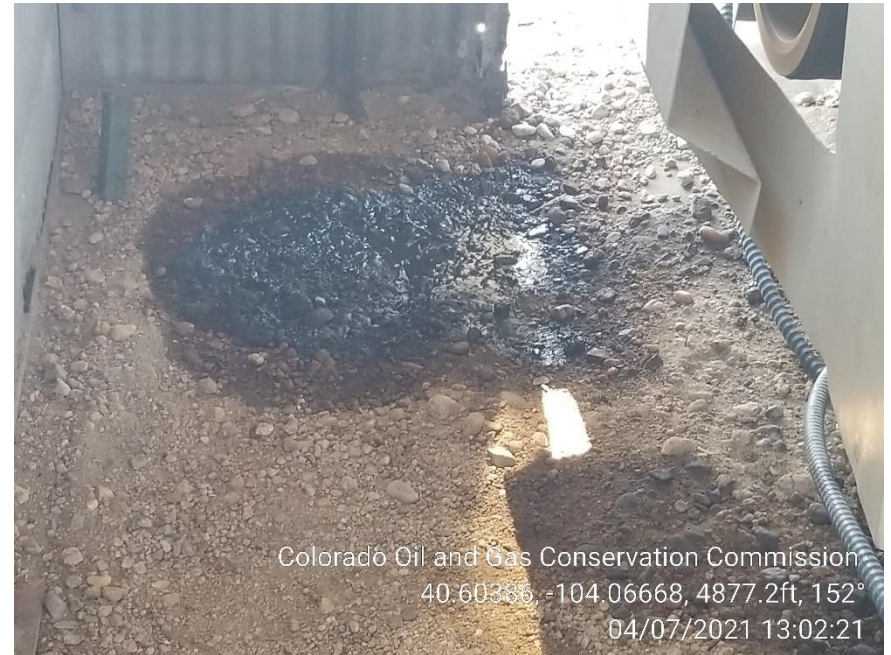
Photo 10 – Stained Soil at Gas Engine
