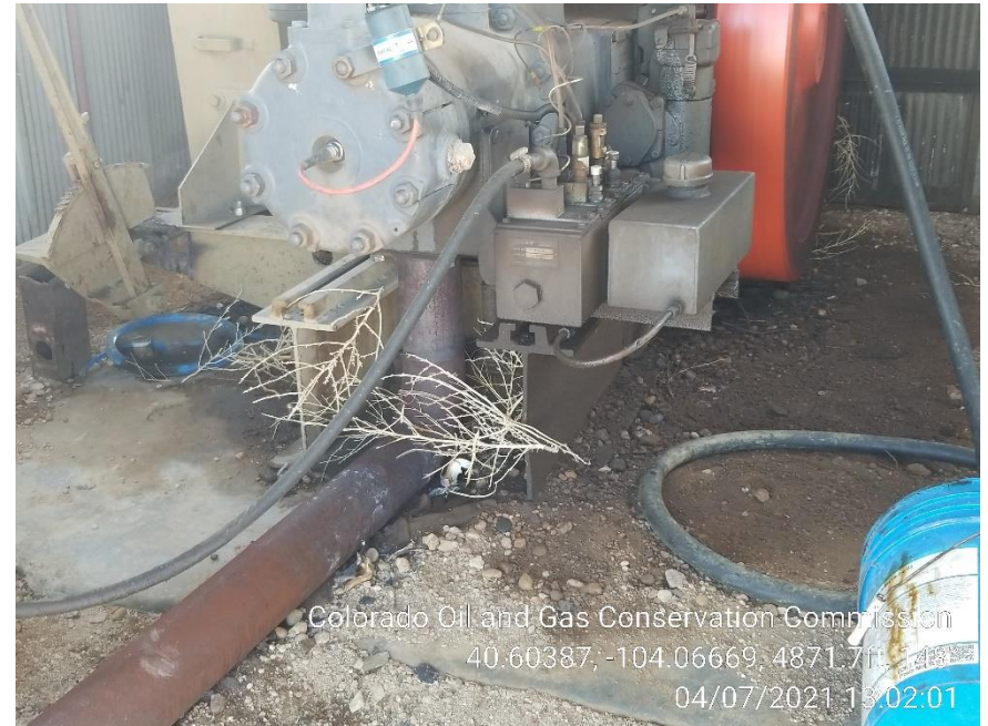
Photo 6 – Stained Soil at Gas Engine
