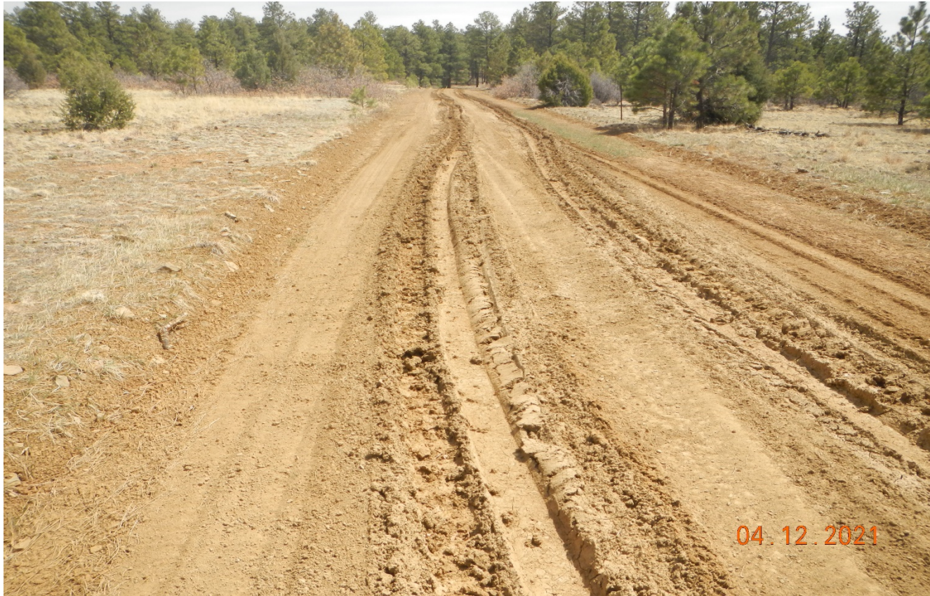
Photo 1. There is vehicle rutting along the access road. Areas of rutting need to be stabilized.
