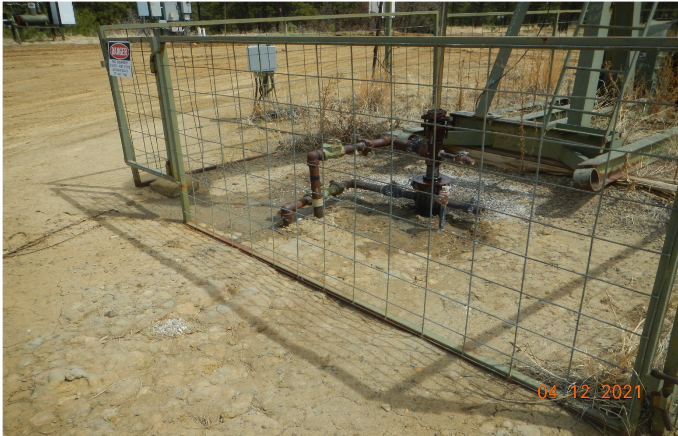
Photo 6. There is slight produced water leaking from the wellhead.
