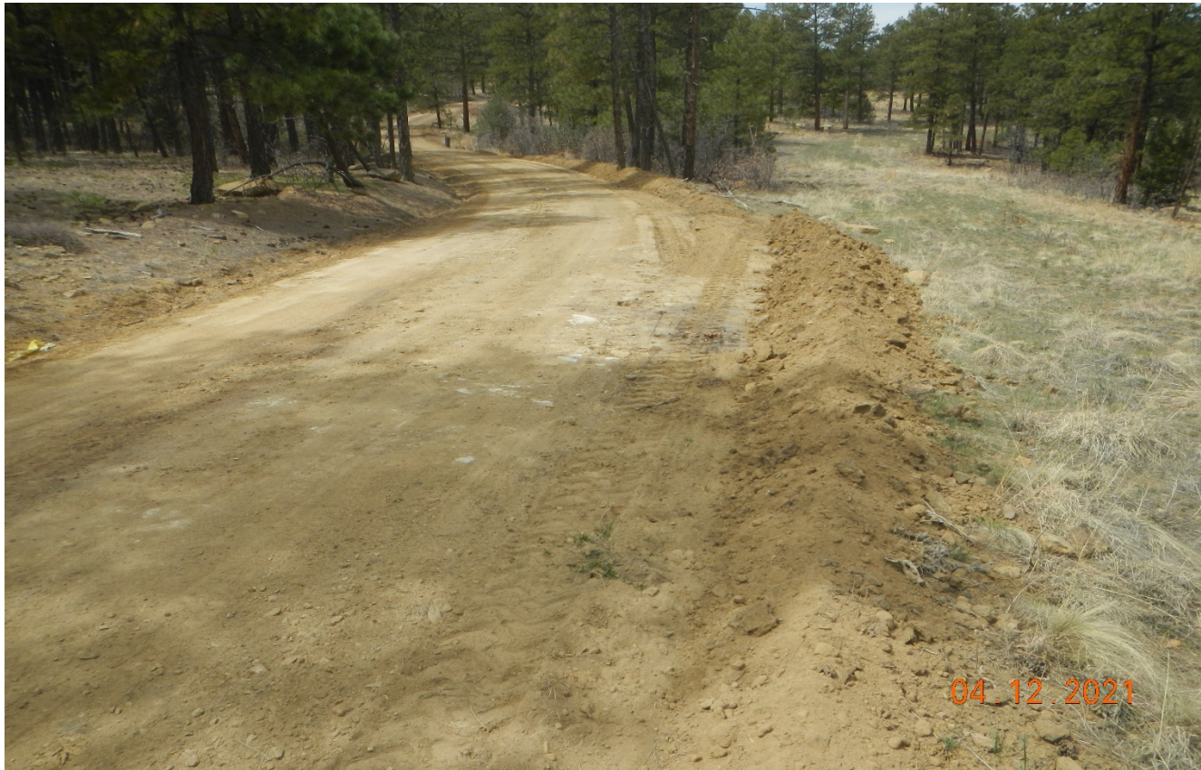
Photo 3. The road which was recently bladed has pushed loose material off the road. There is insufficient stabilization along the road.
