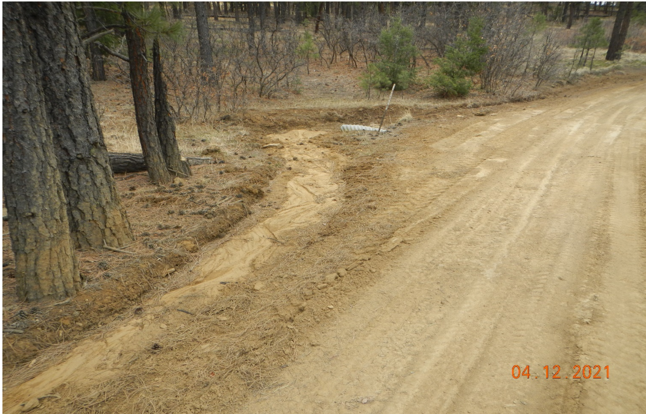
Photo 4. There is sediment accumulation near the culvert which needs to be maintained.
