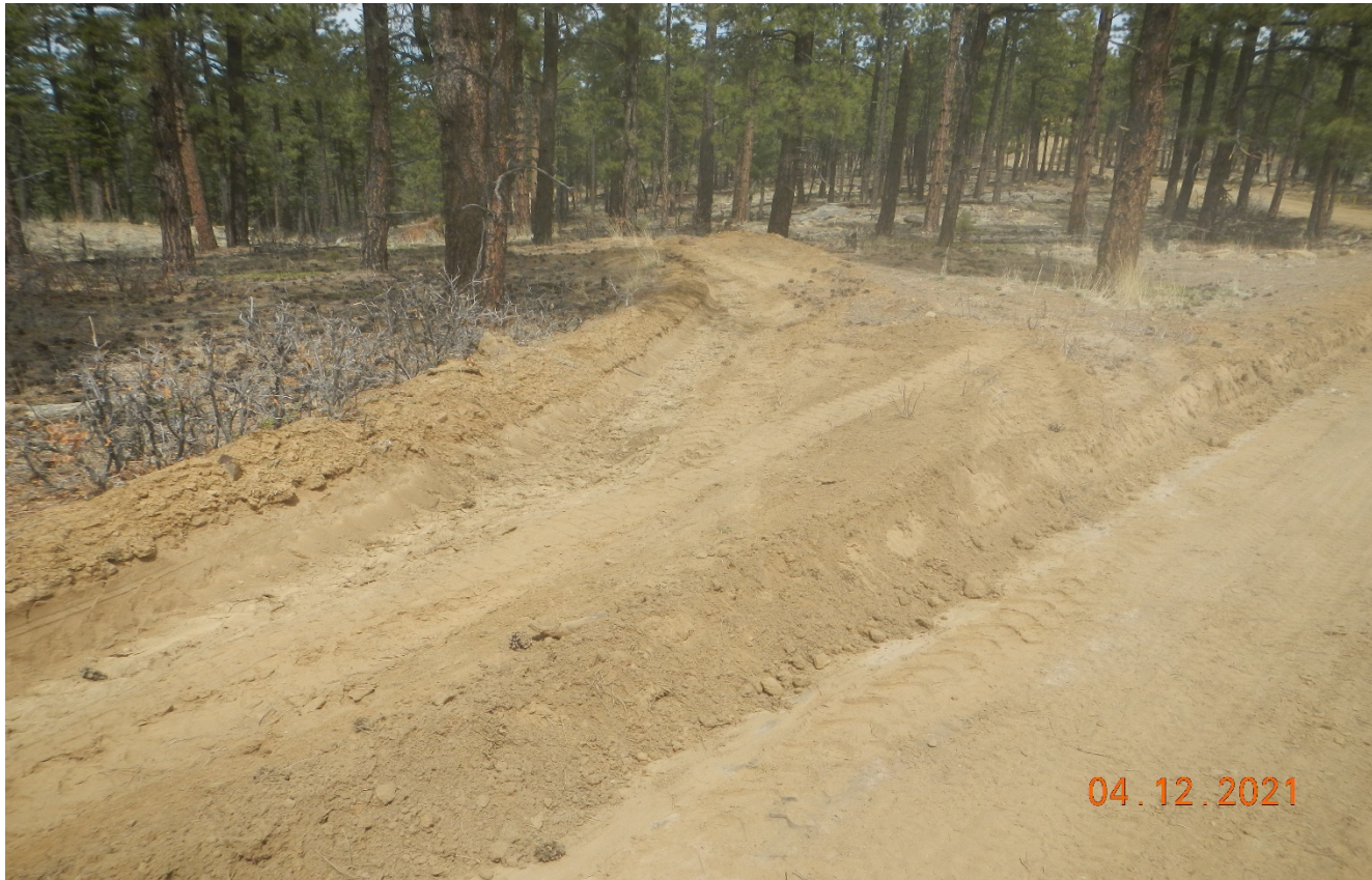
Photo 3. A ditch was bladed to divert stormwater off the road however, BMP's are required to prevent sediment discharge. BMP's such as a sediment trap, rip/rap, check dams need to be installed.
