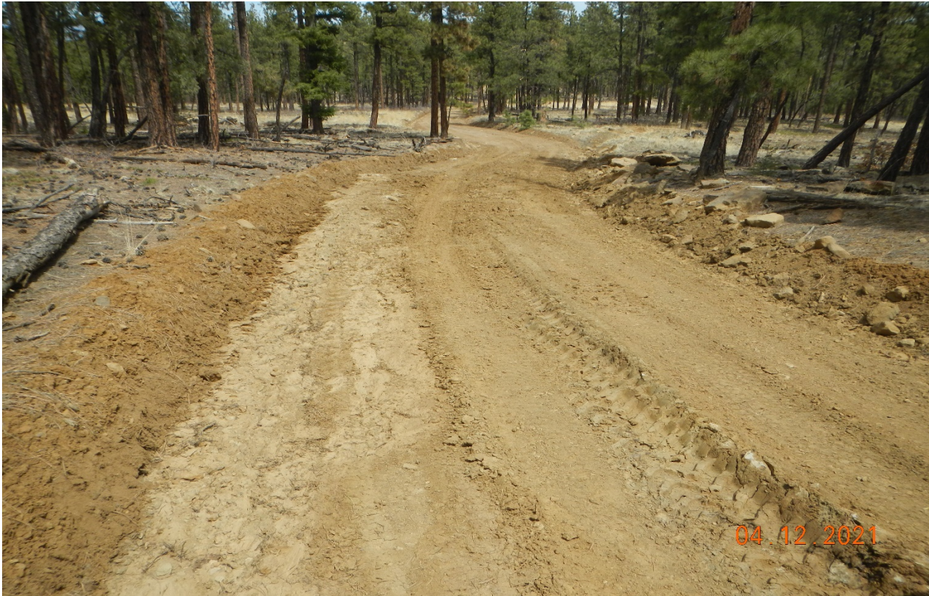
Photo 2. Facing north along the access road. The road is not stabilized
