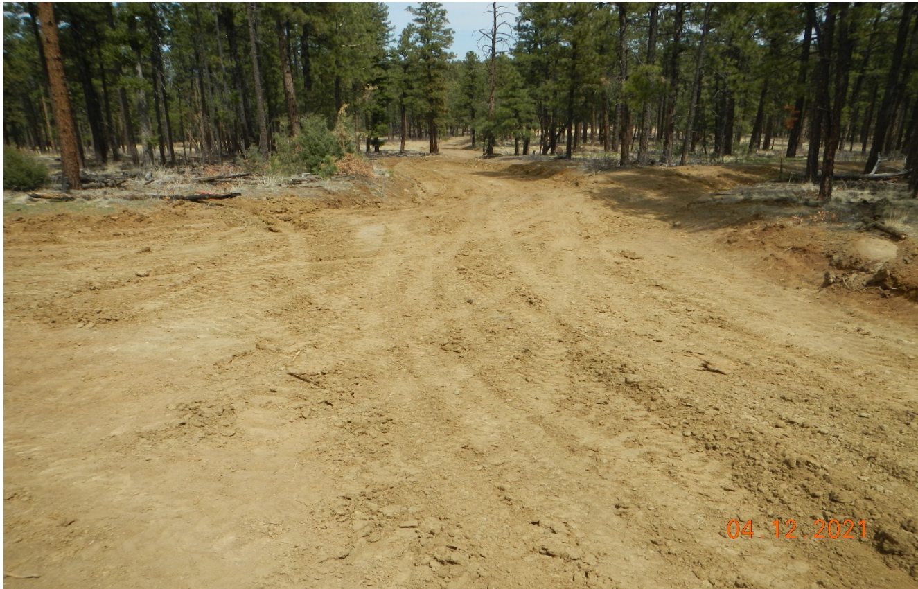
Photo 1. Facing north toward the access road. It appears grading was recently performed however, there is signs of vehicle rutting. The road is not stabilized.
