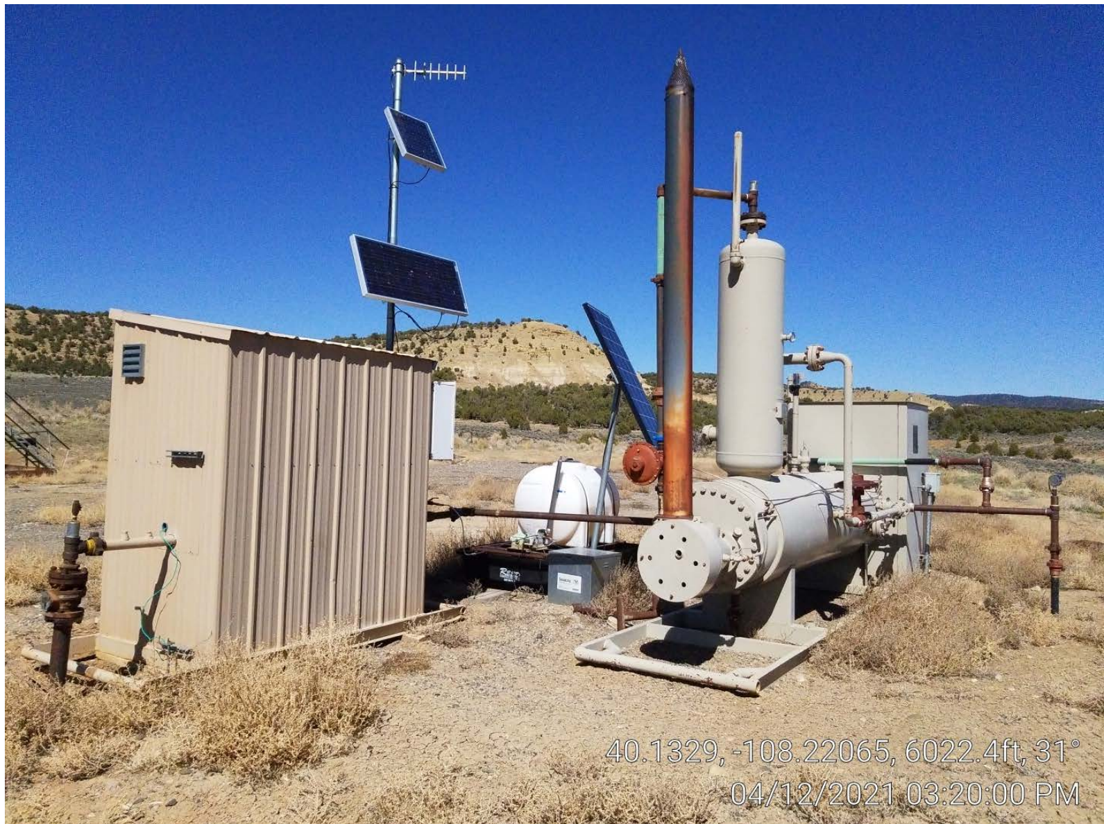
Photo 3. Meter building & separator.
