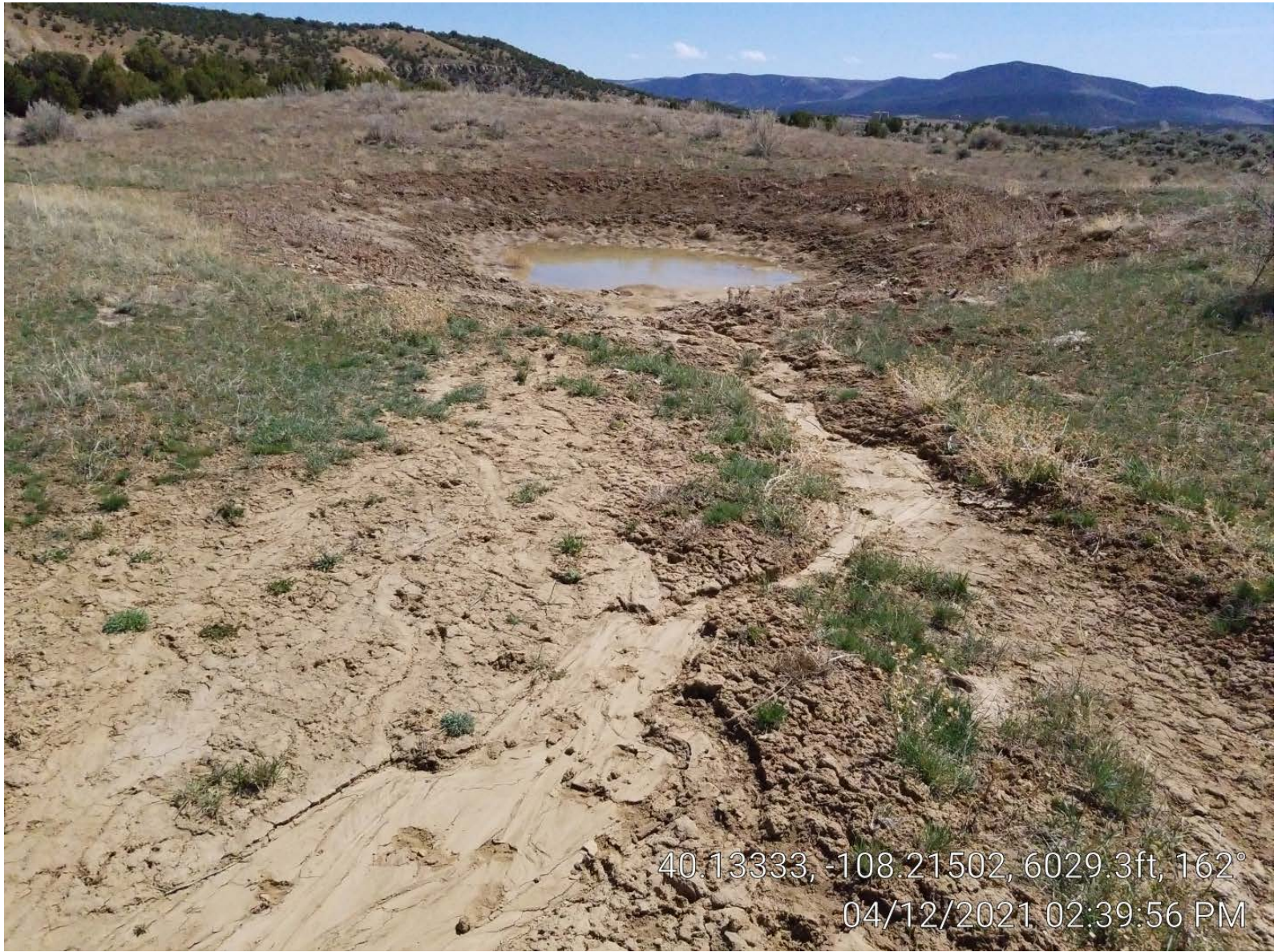
Photo 11. Storm water channels going into retention pond.
