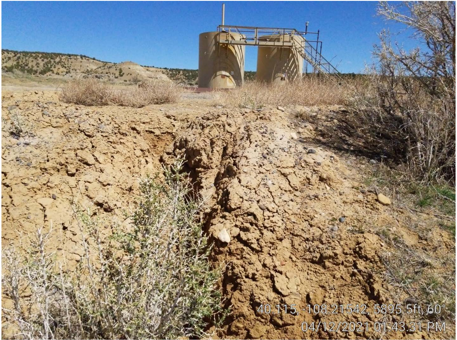
Photo 6. Storm water channel coming off location in retention pond.
