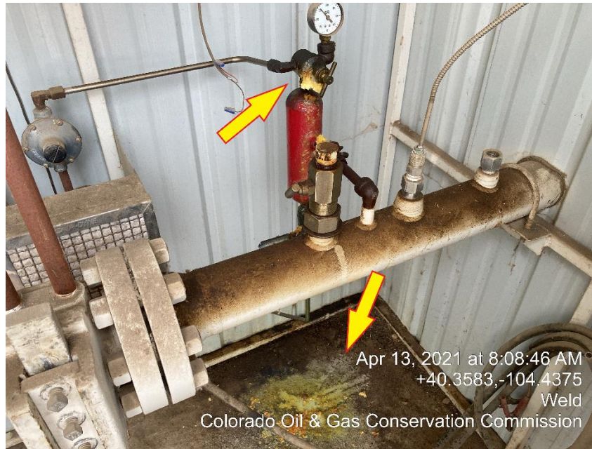
Photo #7 Mechanical Condition/ Oily waste on floor
