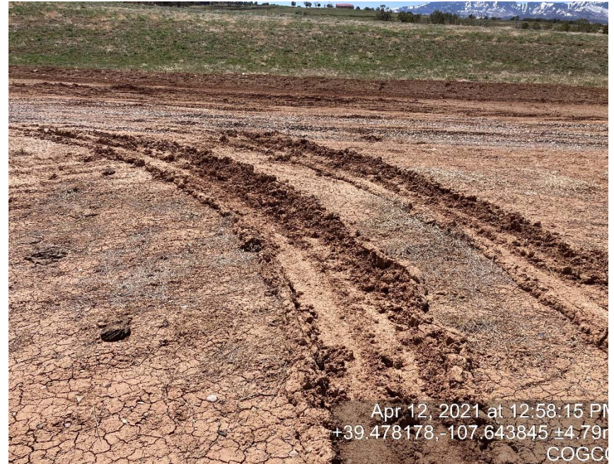
lack of stabilization/compaction
