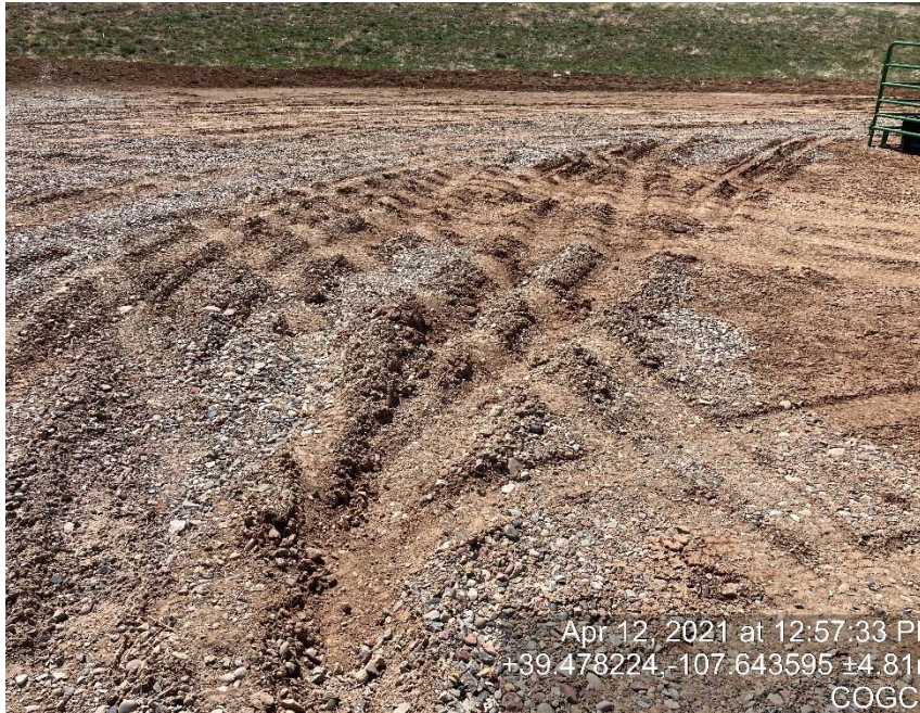
lack of stabilization/compaction
