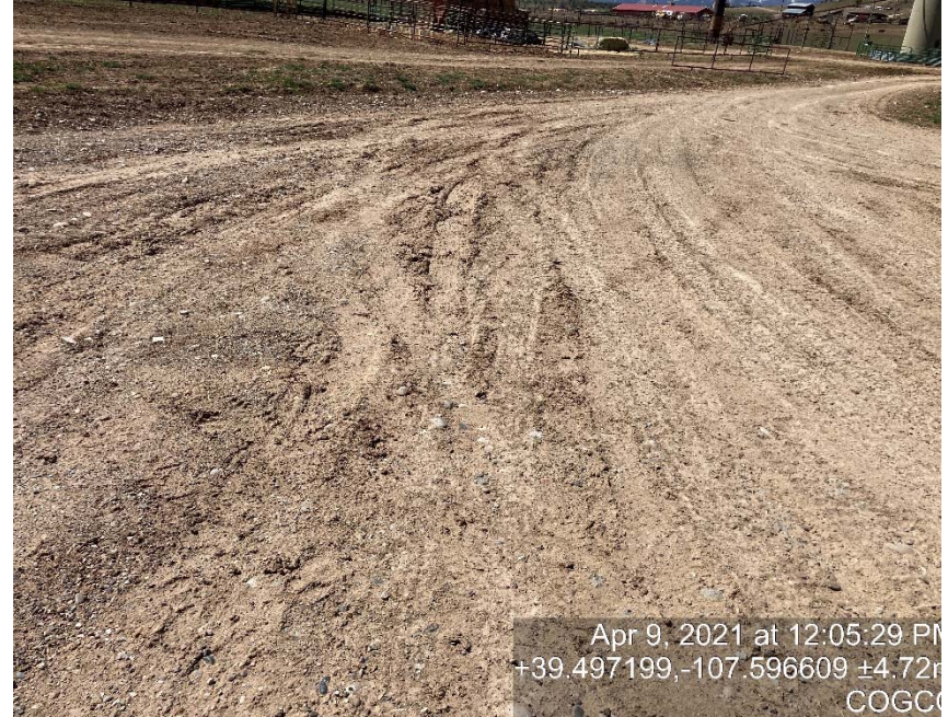
lack of stabilization/compaction
