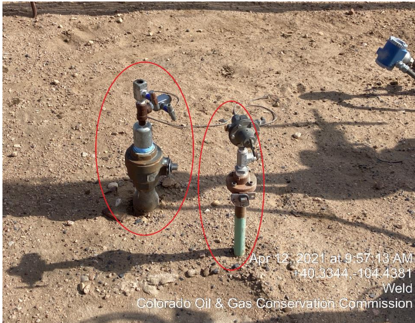
Photo #31 Unmarked Risers
