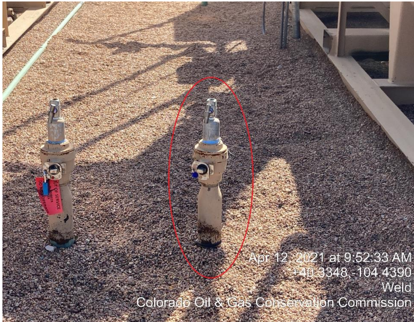
Photo #21 Unmarked Riser
