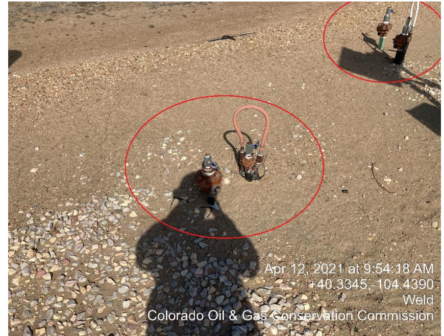
Photo #28 Unmarked Risers
