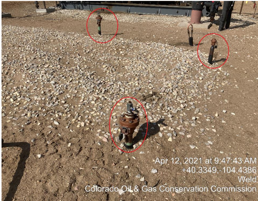
Photo #9 Unmarked Risers
