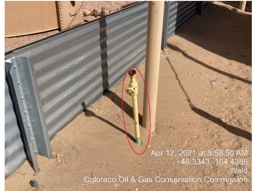
Photo #34 Unmarked Riser
