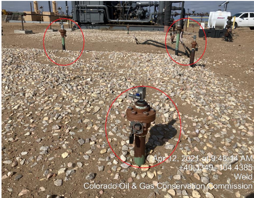
Photo #11 Unmarked Riser
