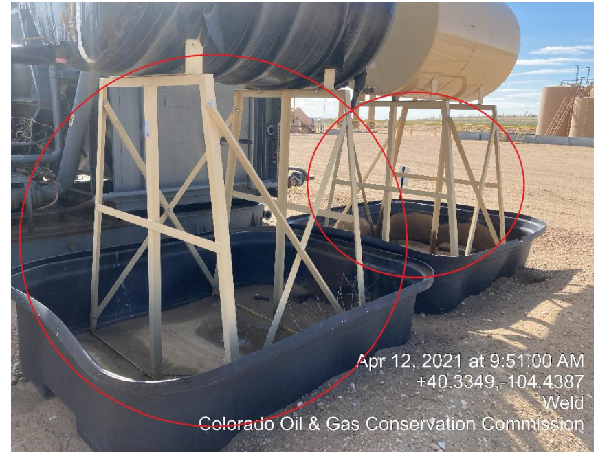
Photo #16 Missing wildlife protective netting
