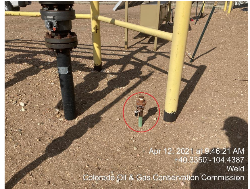
Photo #4 Unmarked Riser
