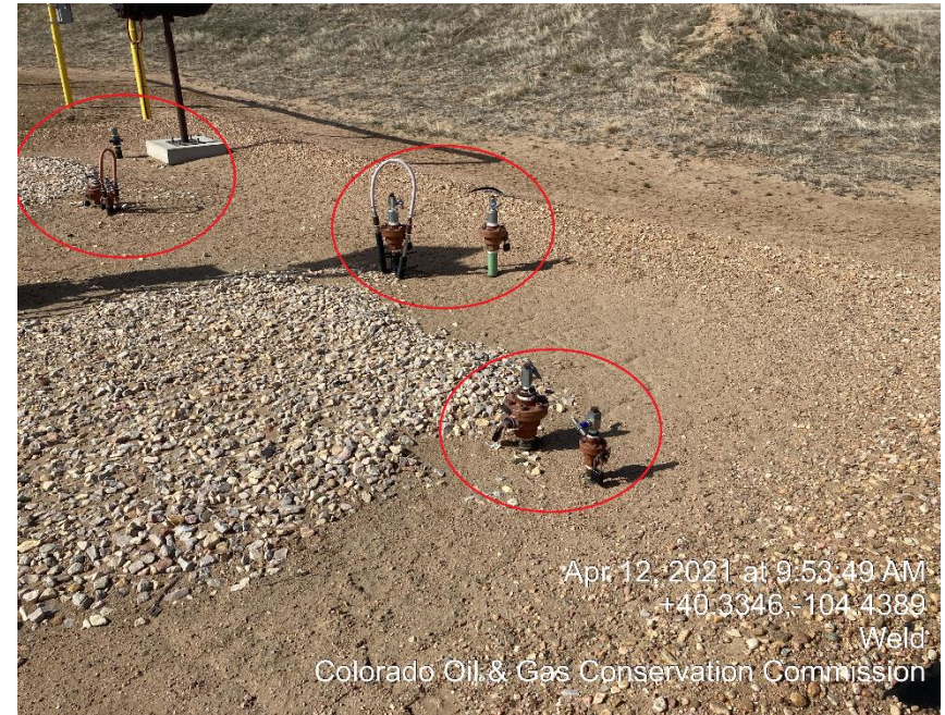
Photo #24 Unmarked Risers
