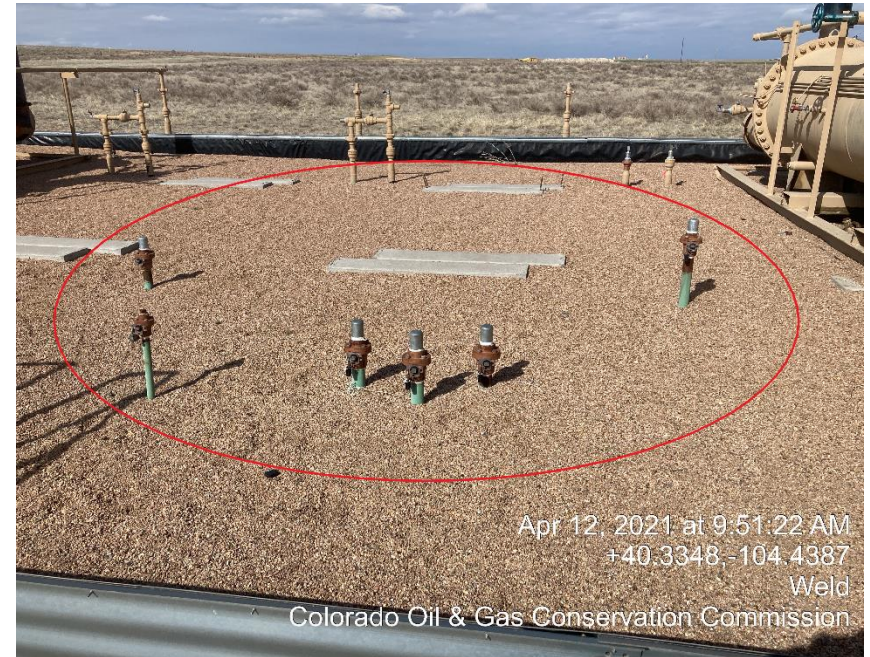
Photo #18 Unmarked Risers
