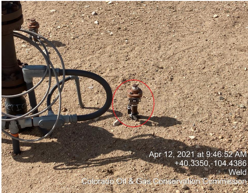
Photo #5 Unmarked Riser
