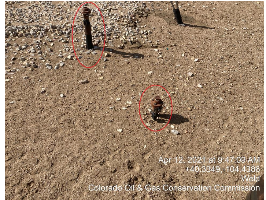
Photo #6 Unmarked Riser
