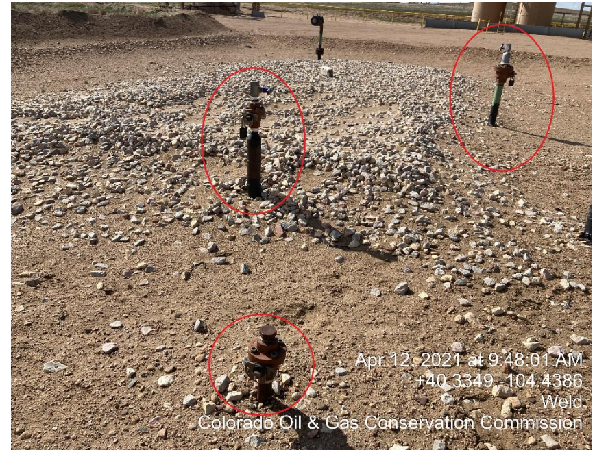
Photo #10 Unmarked Risers
