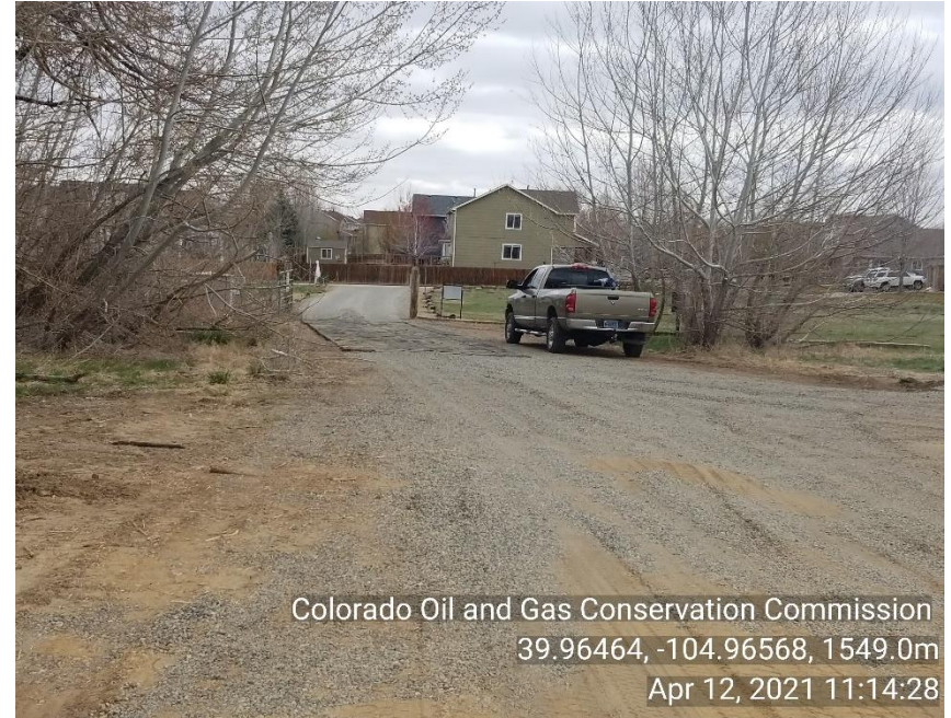
Photo 6 Tracking pad into access road.
