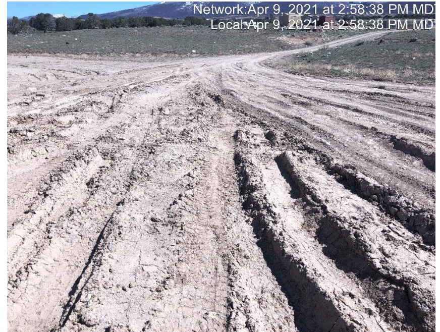
Photo #3449 No form of tracking control at entrance to location.
