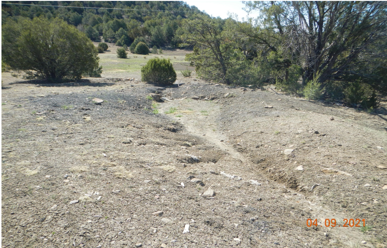
Photo 2. The sediment trap have not been cleaned out and maintained.
