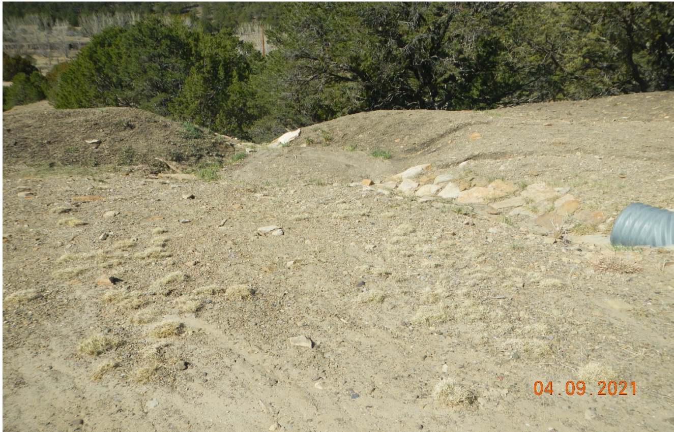
Photo 3. The sediment trap have not been cleaned out and maintained.
