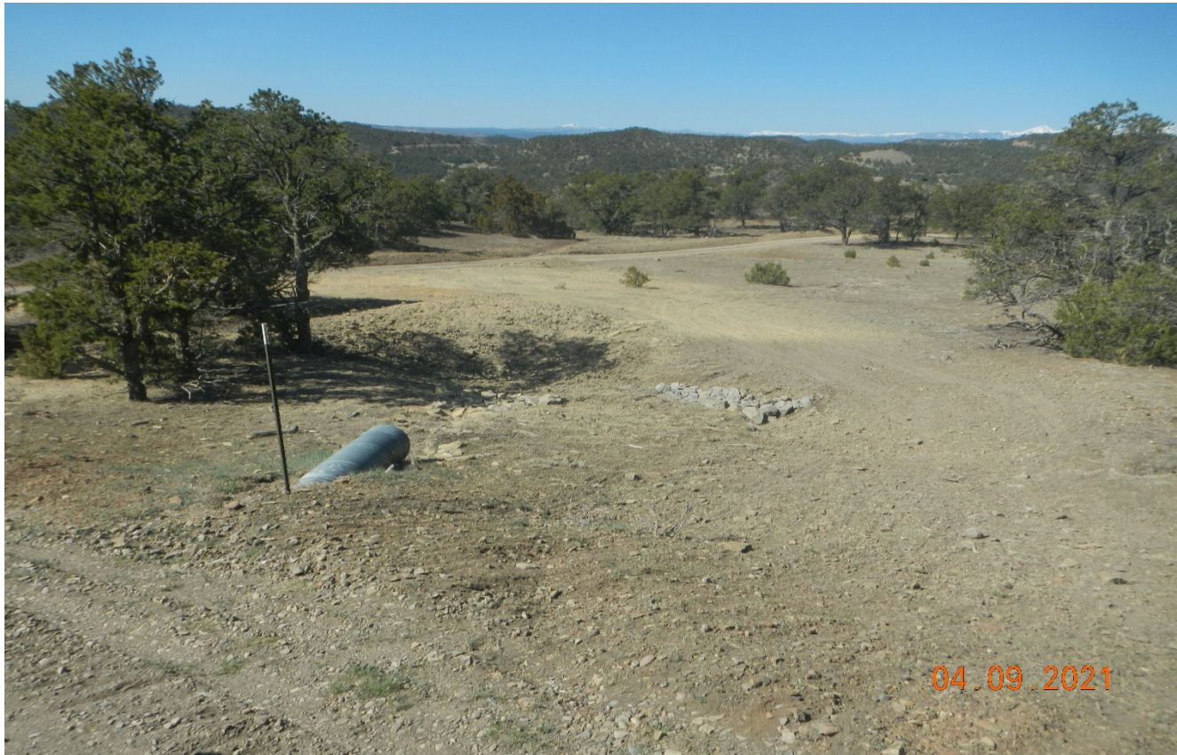
Photo 1. The sediment trap has been maintained along the access road
