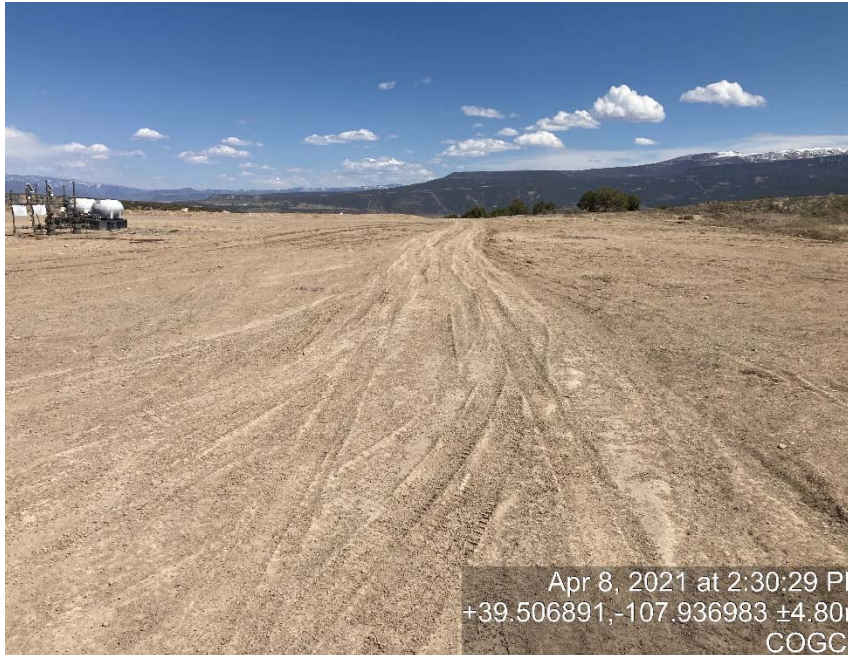
Lack of stabilization/compaction
