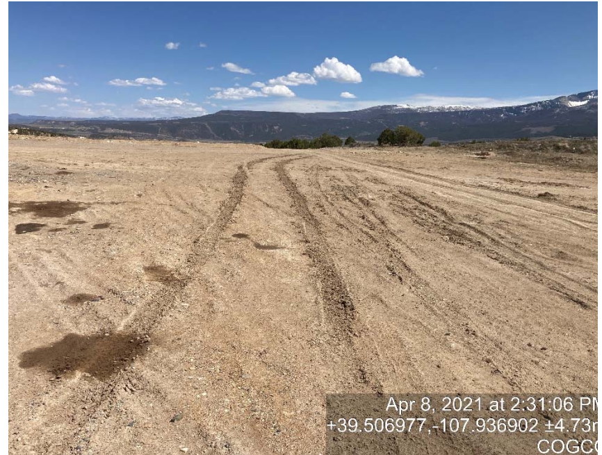
Lack of stabilization/compaction and staining
