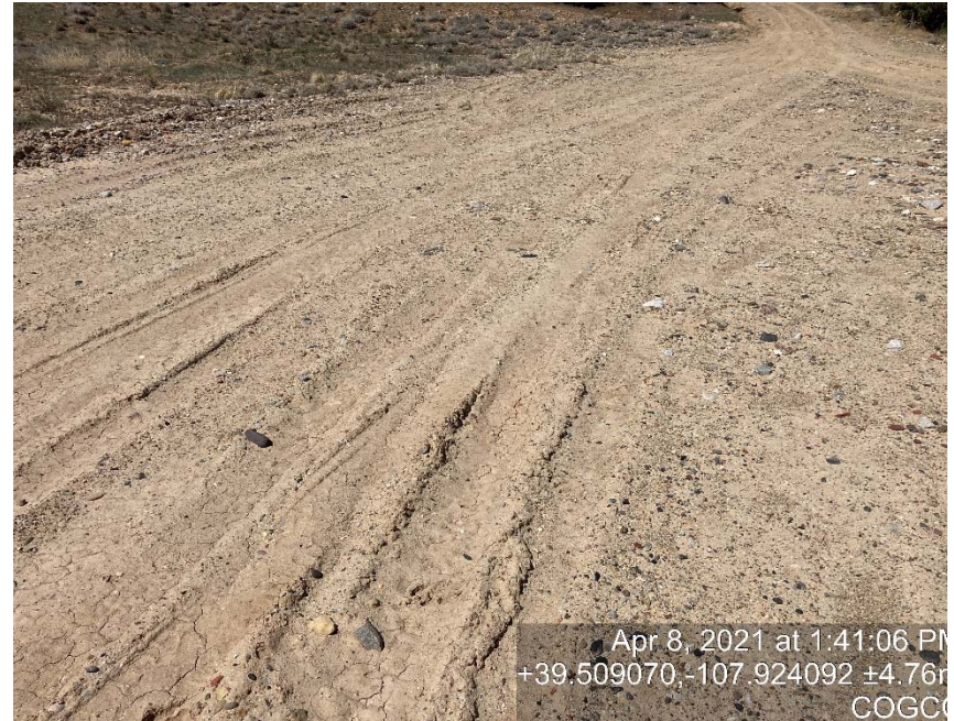
Lack of stabilization/compaction
