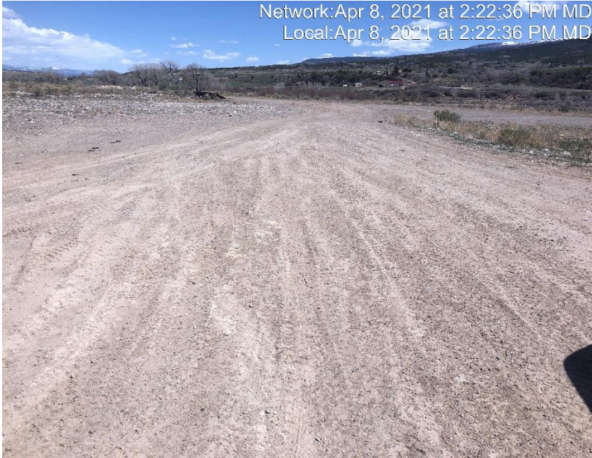
Photo #3431 No form of tracking control at entrance to location.
