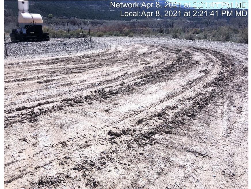
Photo #3430 Location lacks stabilization
