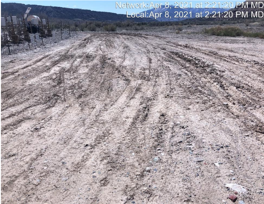
Photo #3429 Location lacks stabilization
