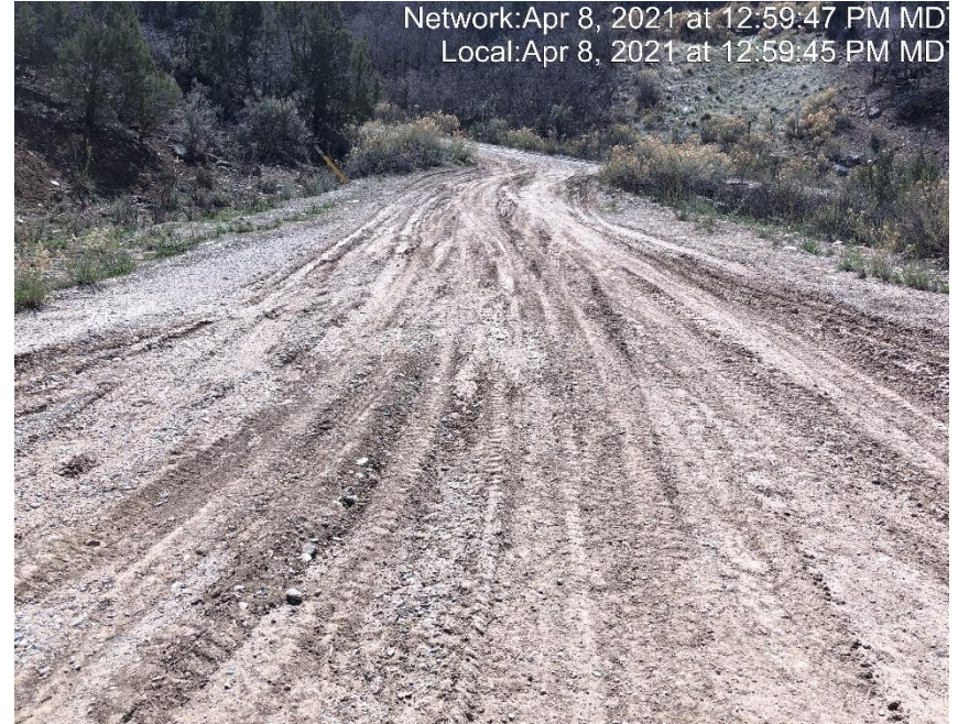
Photo #3426 No form of tracking control at entrance to location.
