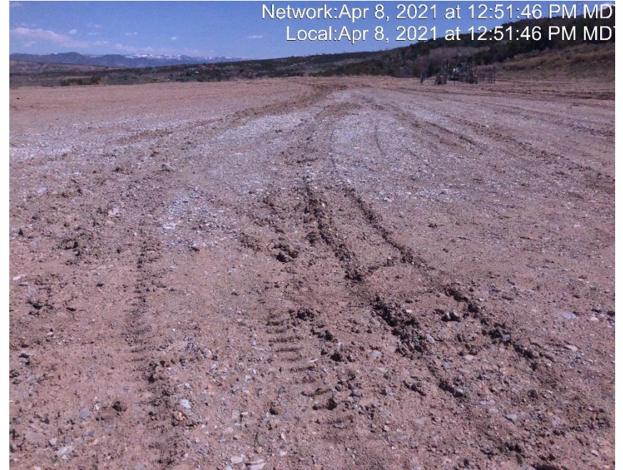
Photo #3413 Location lacks stabilization.
