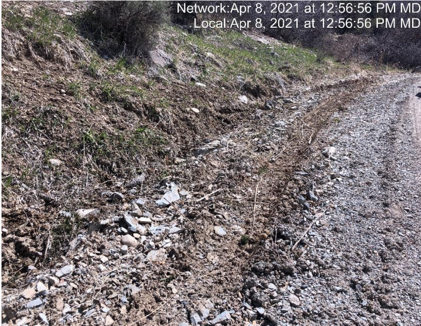
Photo #3421 Storm water is being obstructed.
