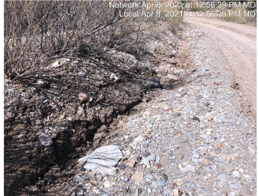
Photo #3419 No velocity checks located in ditch.
