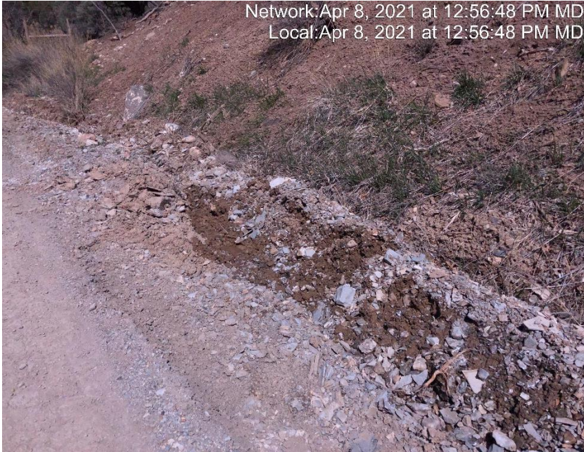
Photo #3420 Storm water is being obstructed.
