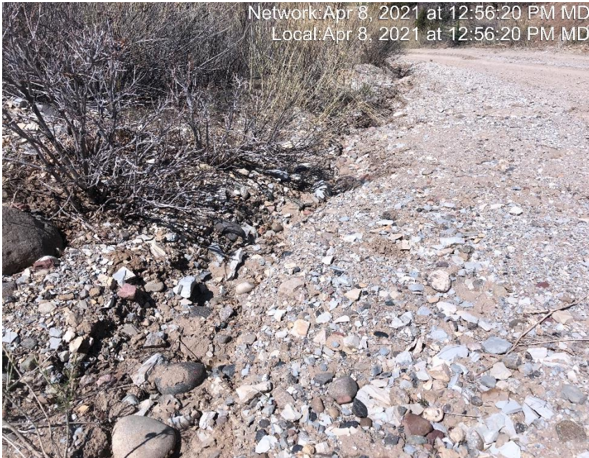
Photo #3418 Rill erosion occurring in ditch.
