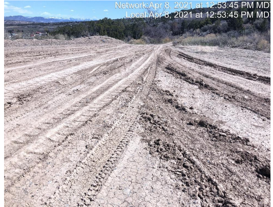
Photo #3417 No form of tracking control at entrance to location.
