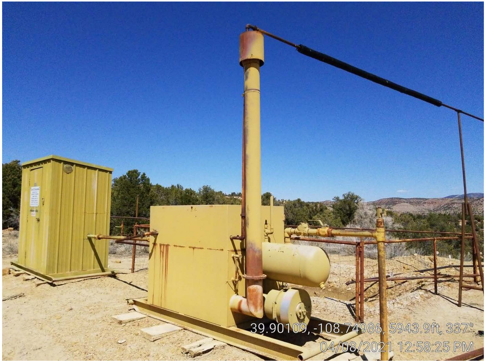
Photo 3. Meter building & separator.
