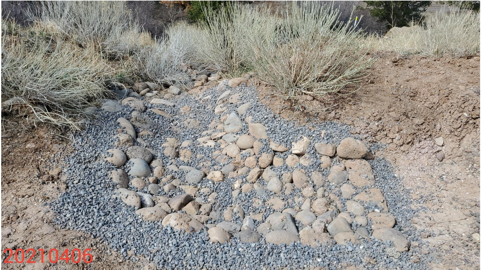
Photo 2: Photo shows control measures to manage stormwater runoff.
