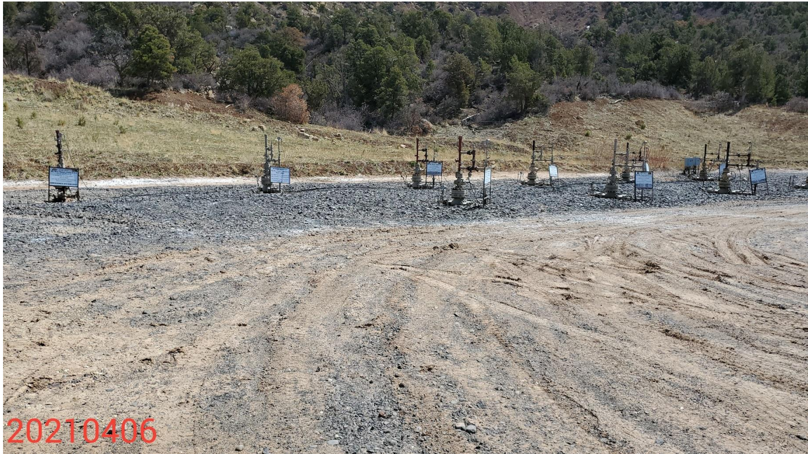
Photo 4: Photo shows producing wells on the Location. Photo also shows gravel has filled with sediment; advise maintenance to ensure pad remains stabilized and to prevent offsite sediment transport.
