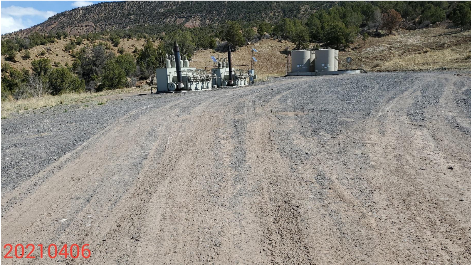
Photo 2: Photo taken from the west end of the Location, facing northeast. Photos 1-2 provide an overview of the Location from northwest to southeast. Photo also shows gravel on production areas is beginning to fill with sediment. Maintenance advised to ensure control measure remains in proper functioning condition to stabilize Location and prevent offsite sediment transport.
