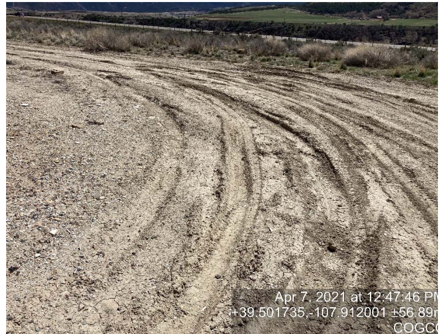
Lack of stabilization/compaction
