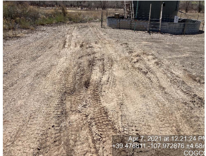
Lack of stabilization/compaction
