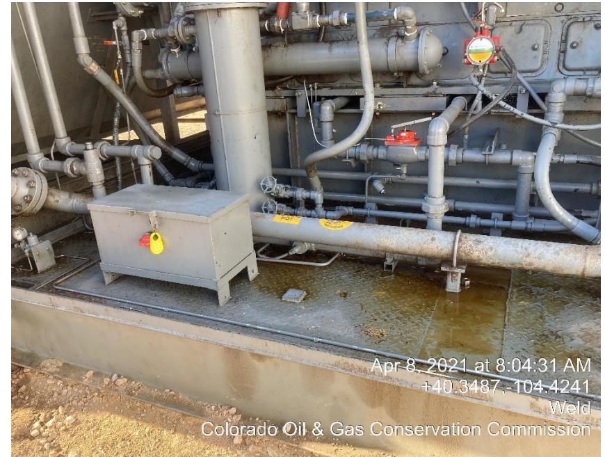
Photo #8 Mechanical conditions/ Oily Waste
