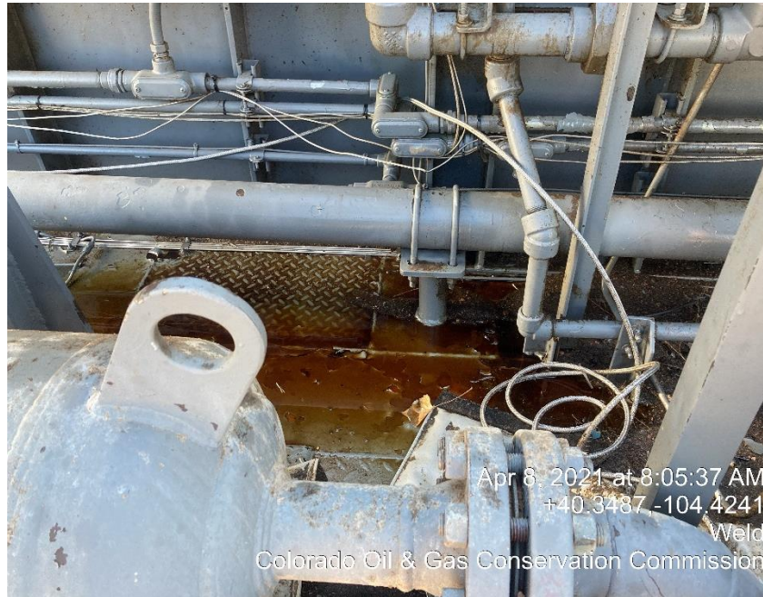
Photo #11 Mechanical conditions/ Oily Waste
